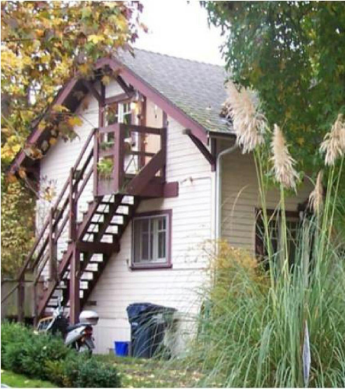
Secondary Dwelling Unit
