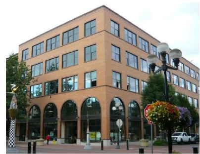
Beam Development rehabilitated this key building in downtown with City Assistance-- fostering incubator place in a high profile, newly refurbished space.
