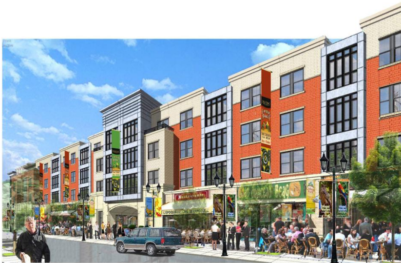
BUILDING 2 FROM MOUNT HOPE AVE
