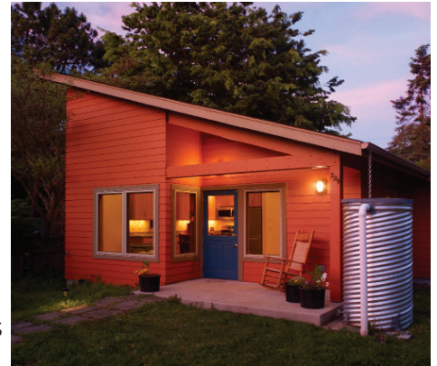
Photo Credit: Rainbow Valley Design and Construction
