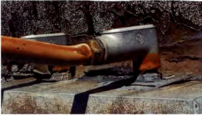
Deteriorated weather-proofing.
