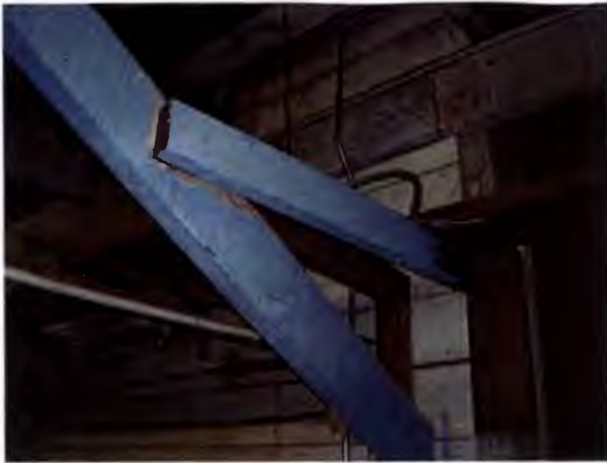
Alteration to structural framing.
