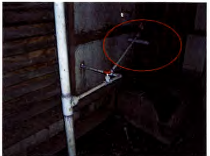
Drain of utility sink, drains to ground.
