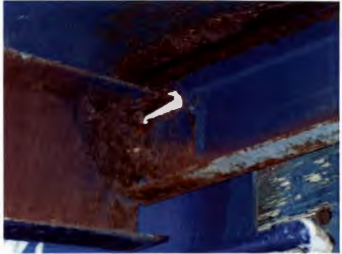
Structural support below metal bleacher section.
