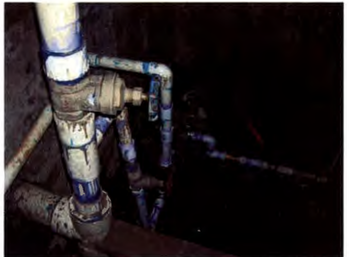
Plumbing cross connections and improper pipe material.
