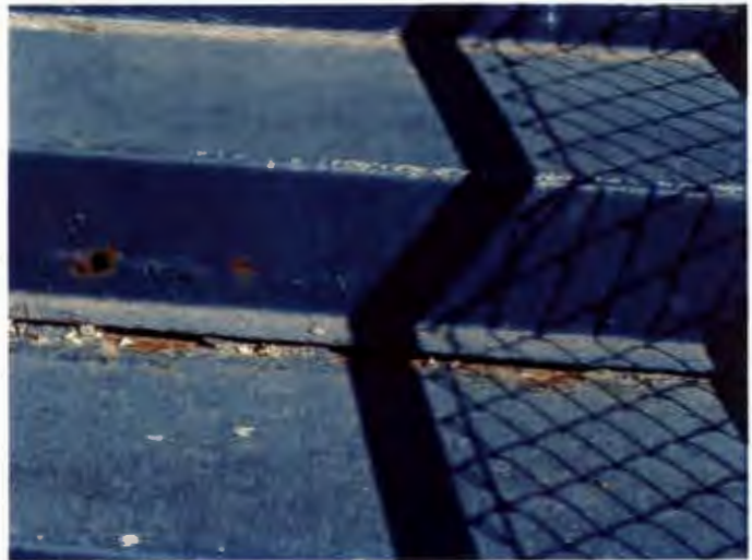
Metal stairs to raised bleacher seats.
