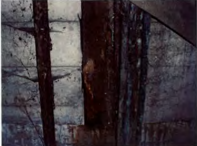
Roof downspout drains to grade along foundation. Visible signs of dry rot.
