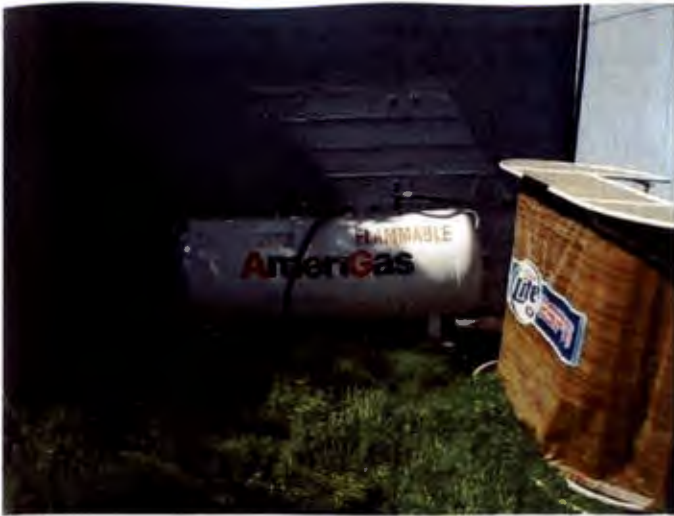
Propane accessible and open to the public.
