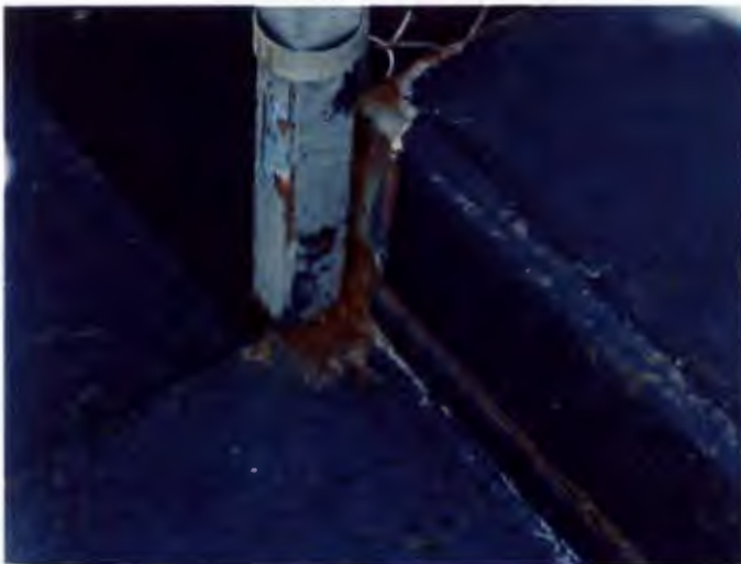
Metal stairs and hand rails.
