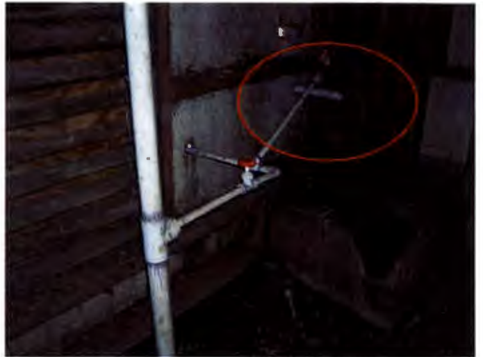
Drain of utility sink, drains to ground.
