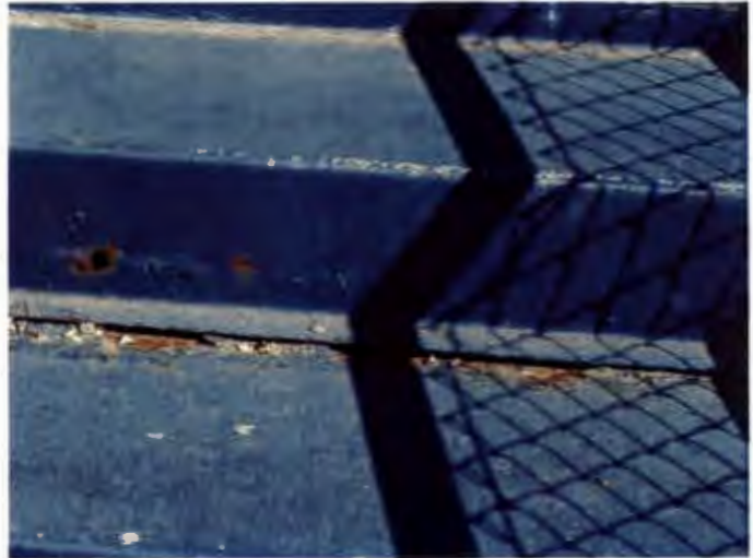
Metal stairs to raised bleacher seats.
