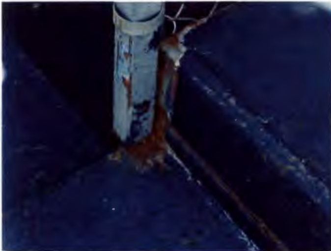
Metal stairs and hand rails.
