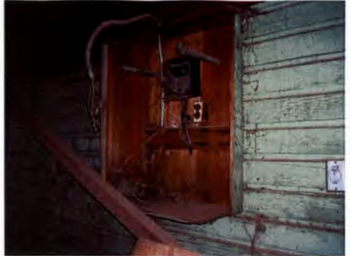
Exposed wiring.
