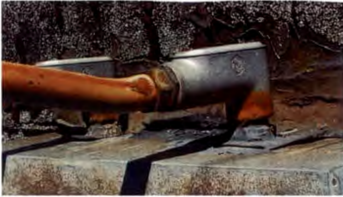
Deteriorated weather-proofing.
