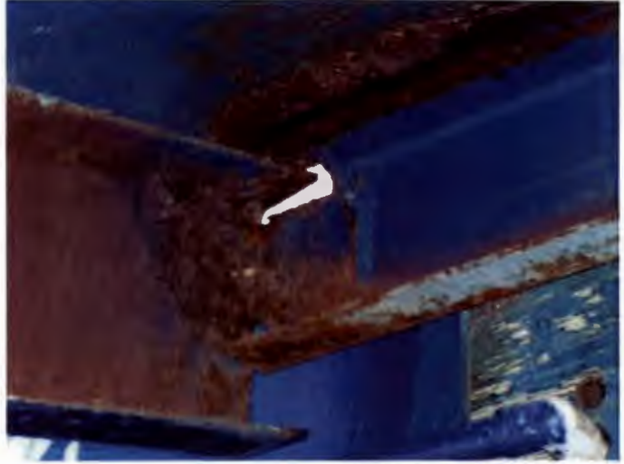
Structural support below metal bleacher section.
