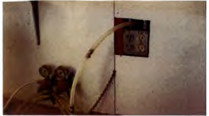
Carbonation tubing in outlet wiring chase.
