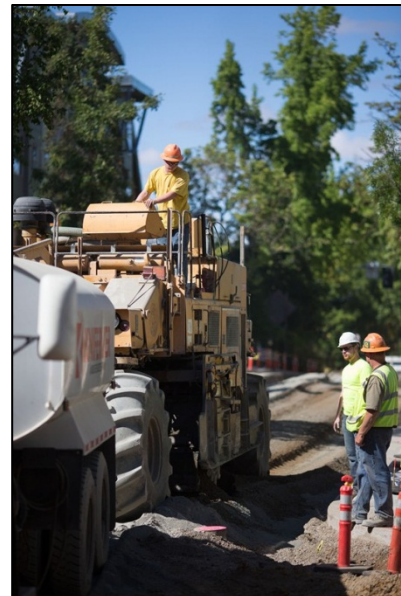
In-place recycling on Alder Street
