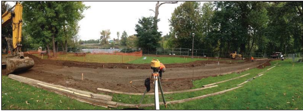
Reconstruction of South Bank Path
