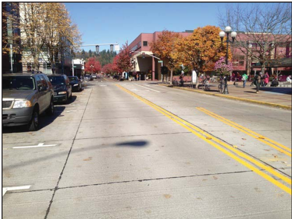
Olive Street post-construction – New concrete pavement at the LTD station
