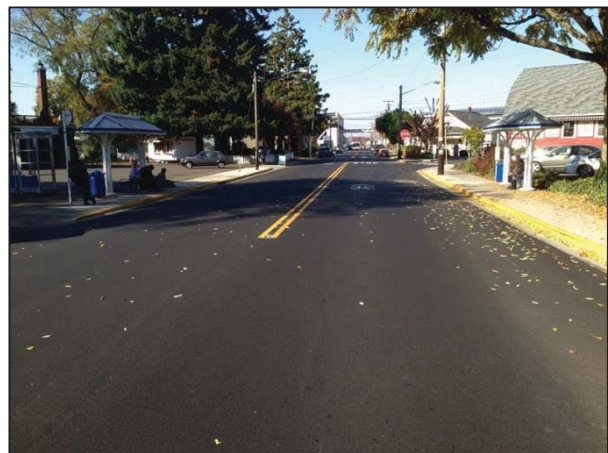
Blair Boulevard post-construction
