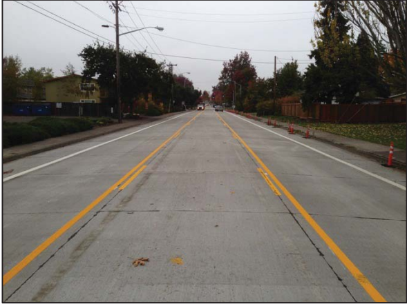
18th Avenue post-construction
