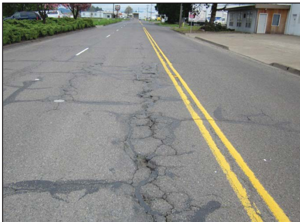
5th Avenue pre-construction
