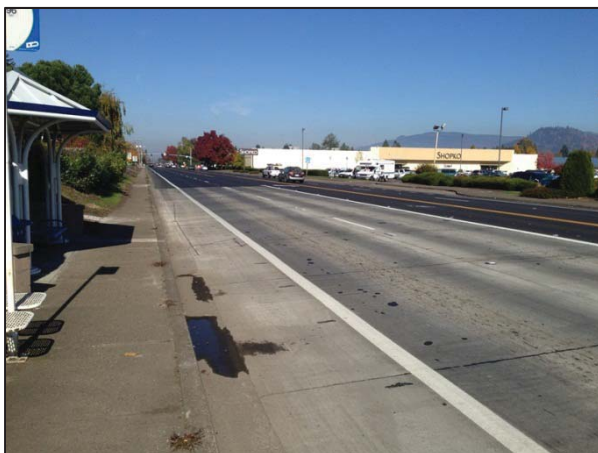
Coburg Road post-construction (concrete intersection paving)
