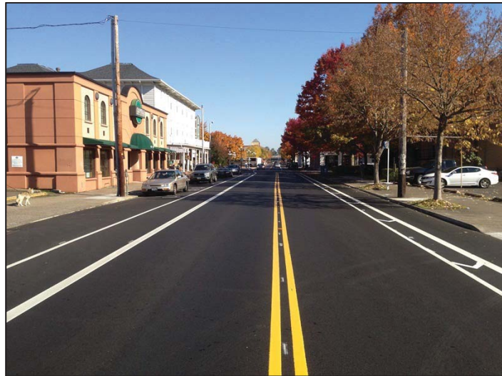
5th Avenue post-construction
