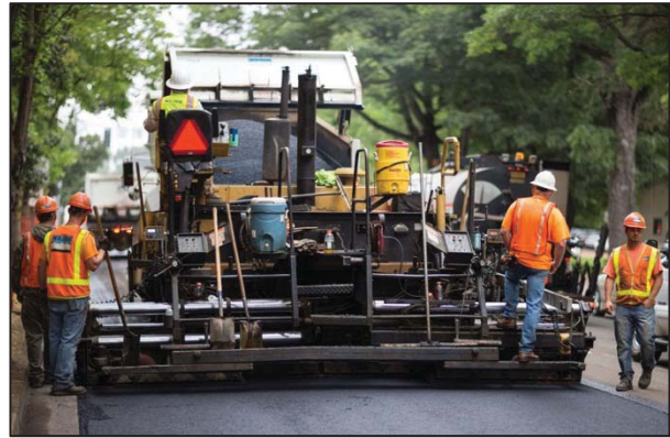
Paving on Hilyard Street
