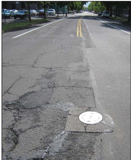
5th Avenue pre-construction
