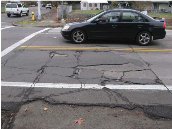
18th Avenue pre-construction
