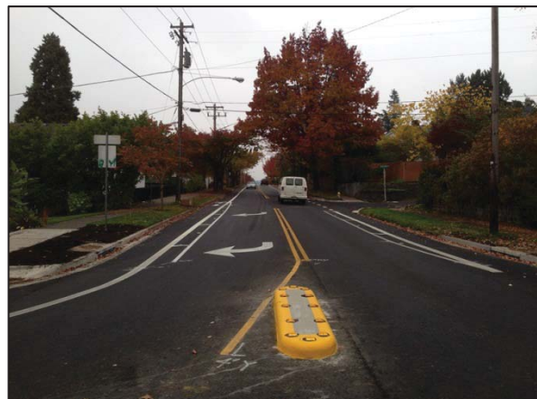
Willamette Street post-construction
