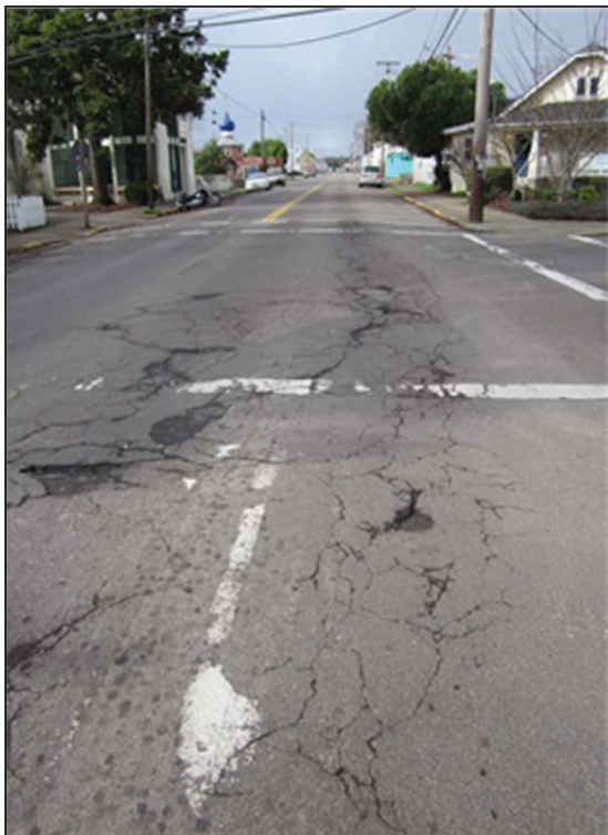
Blair Boulevard pre-construction
