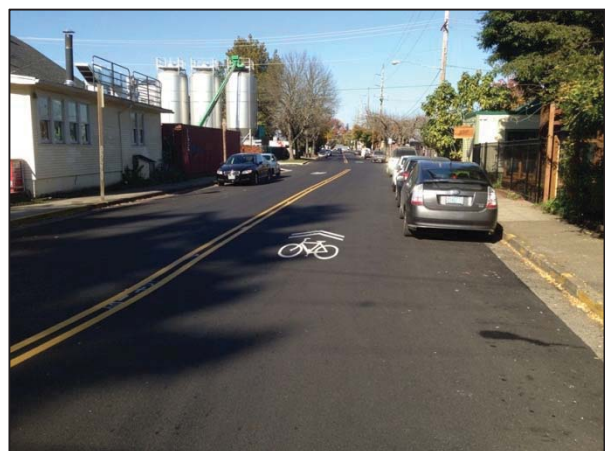
Van Buren Street post-construction
