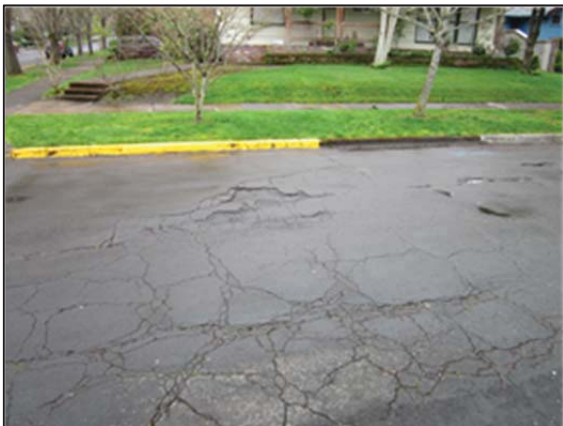
Alder Street pre-construction
