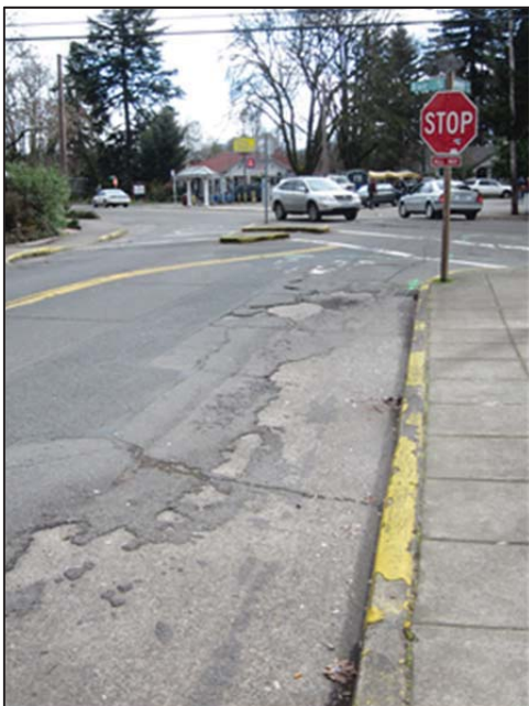
Van Buren Street pre-construction
