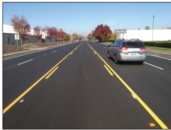
Coburg Road post-construction
