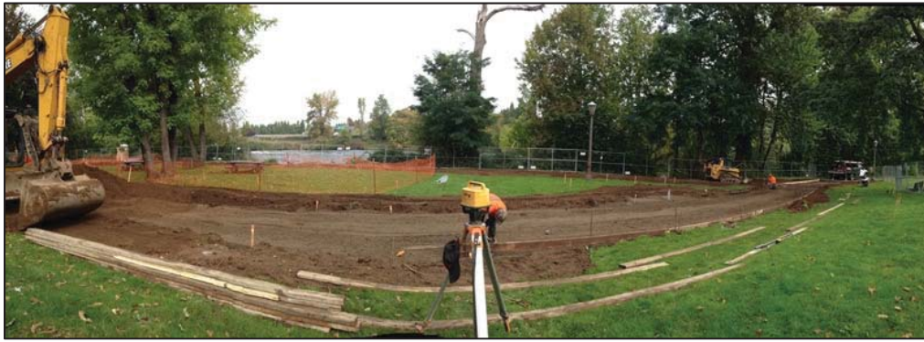
Reconstruction of South Bank Path
