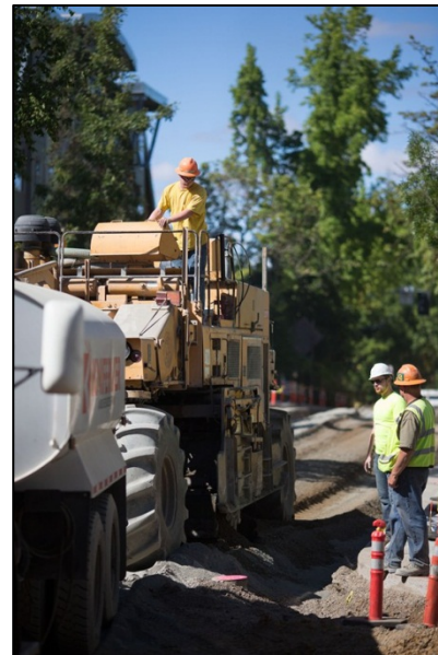
In-place recycling on Alder Street
