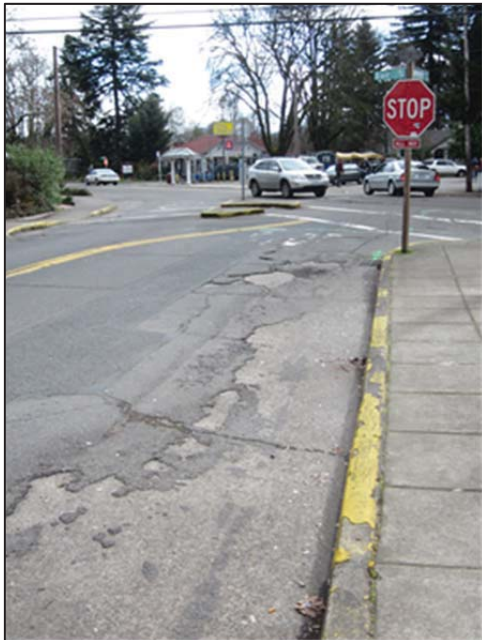
Van Buren Street pre-construction
