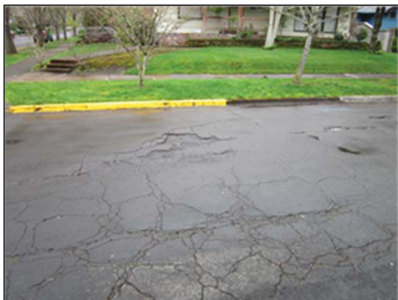
Alder Street pre-construction
