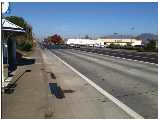
Coburg Road post-construction (concrete intersection paving)
