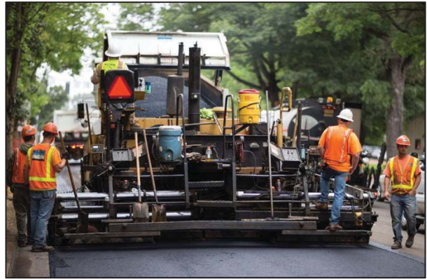
Paving on Hilyard Street
