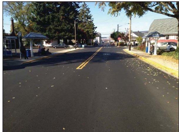
Blair Boulevard post-construction
