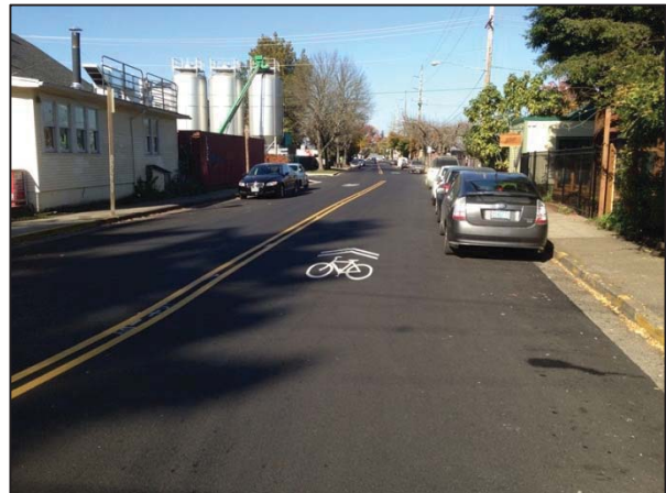
Van Buren Street post-construction
