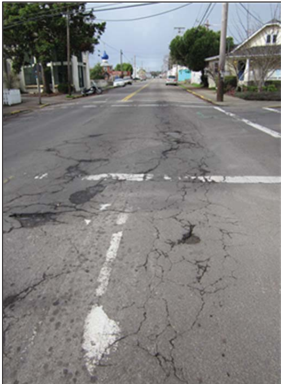
Blair Boulevard pre-construction
