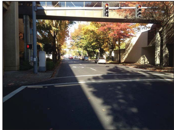
Hilyard Street post-construction
