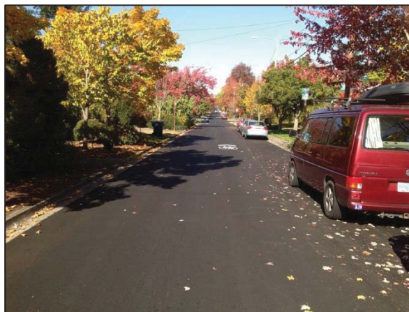
Alder Street post-construction
