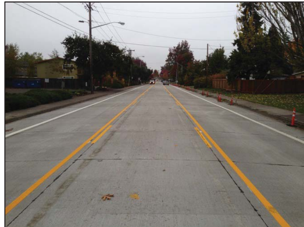
18th Avenue post-construction
