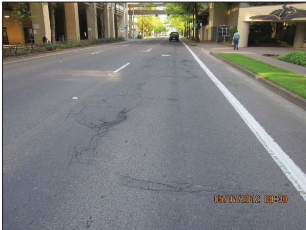
Hilyard Street pre-construction
