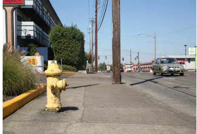
Example of utility conflicts in sidewalk.
