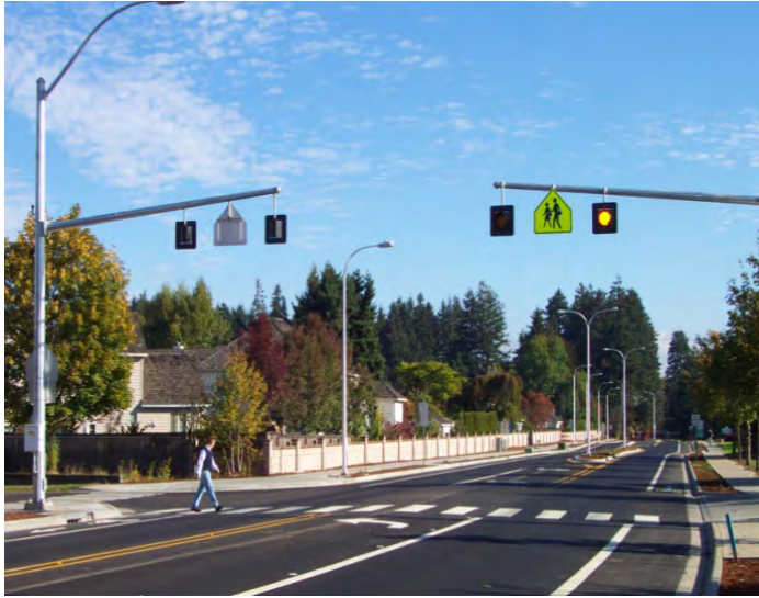
Figure 16 – Overhead Flashing Beacon
