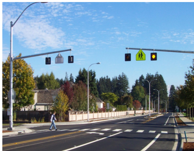
Overhead flashing beacons inform drivers that pedestrians are crossing the road.
