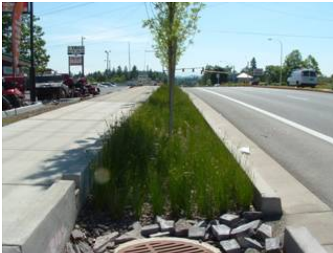
Example of bioswales (Source: OTAK)
