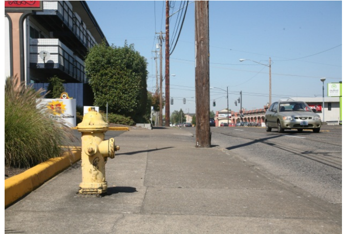
Example of utility conflicts in sidewalk.
