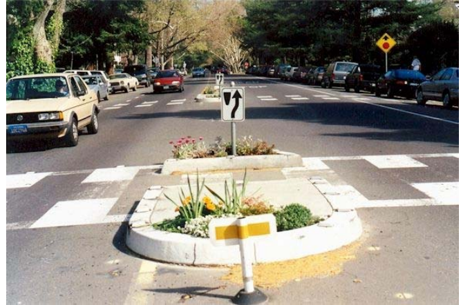
Median pedestrian crossing refuges provide a waiting area for a two-stage pedestrian crossing.
