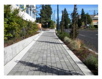
Example of permeable paving.
