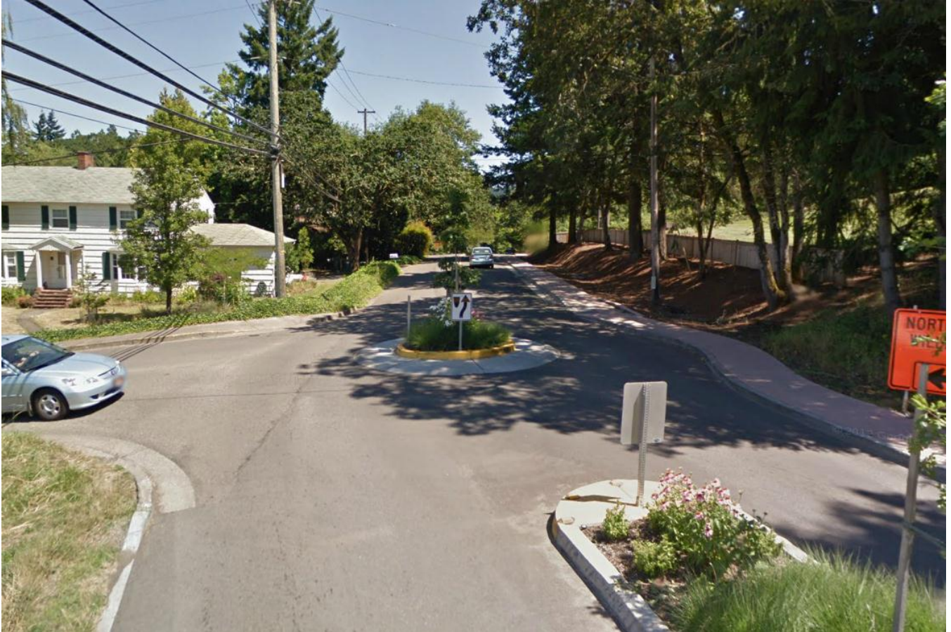
Crest Drive – Lincoln Street Traffic Circle
