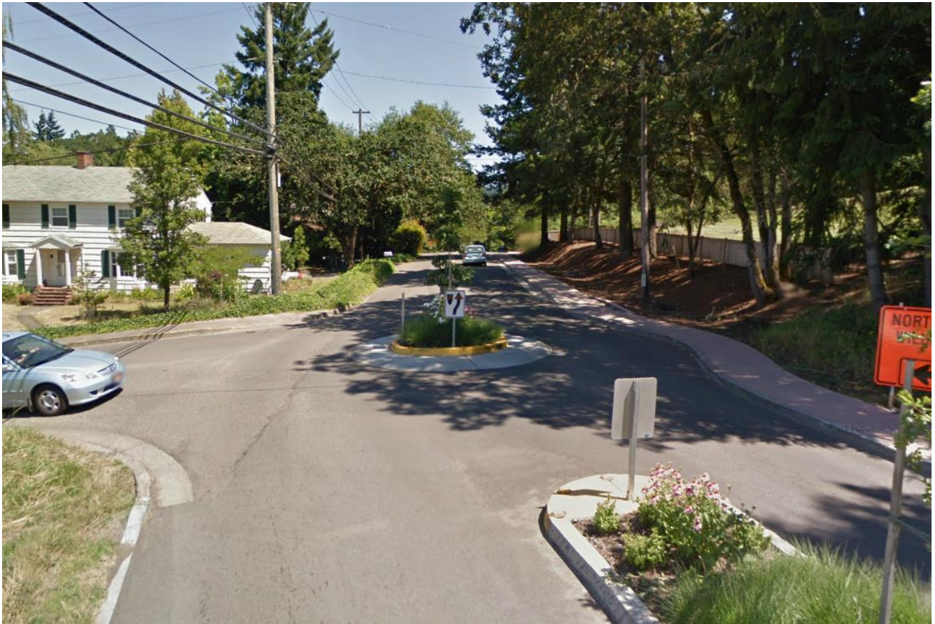
Crest Drive – Lincoln Street Traffic Circle
