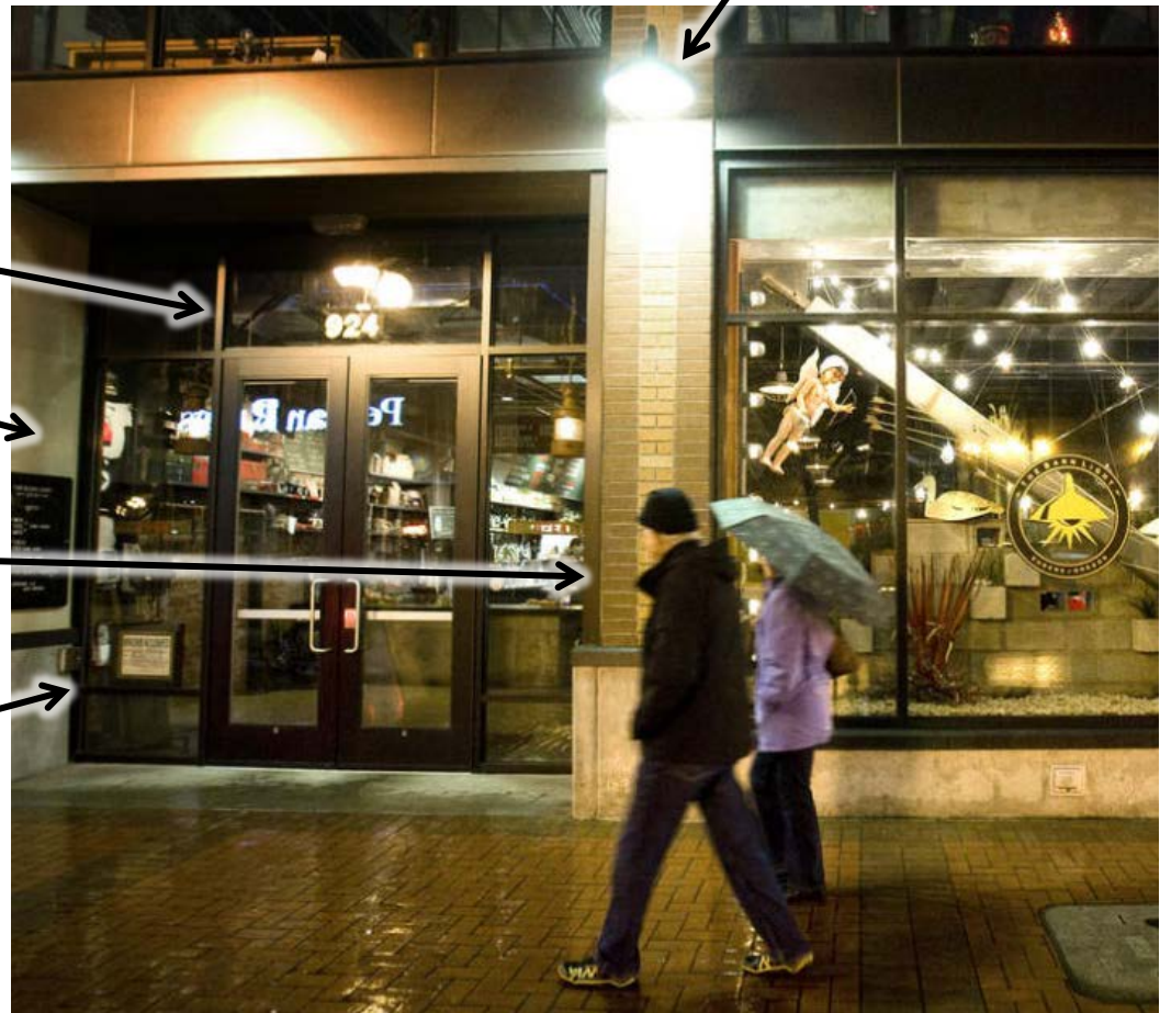
Center Court Building – Broadway Commerce Center
