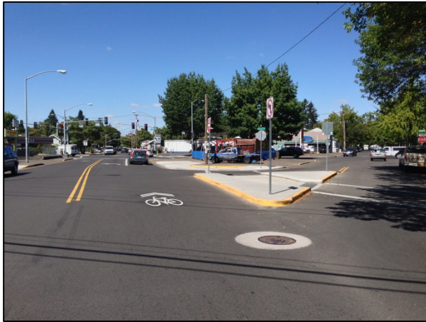
Blair Avenue Streetscape Sidewalk, curb ramps, and crossings
