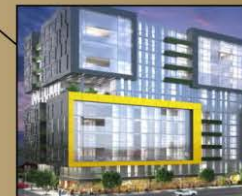
The HUB (under construction)
