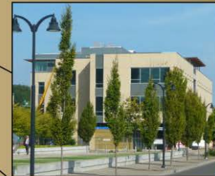
Northwestto Juo Community Credit Union (NWCCU) (under construction)
