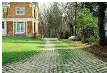
EC 9.3868(8)(d)7. Pervious Paving
