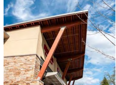
EC 9.3858(8)(b)2.a.Revealed Structural Elements
