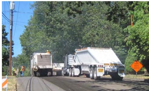
Removing top layers of pavement on 40<sup>th</sup> Avenue for inlay treatment
