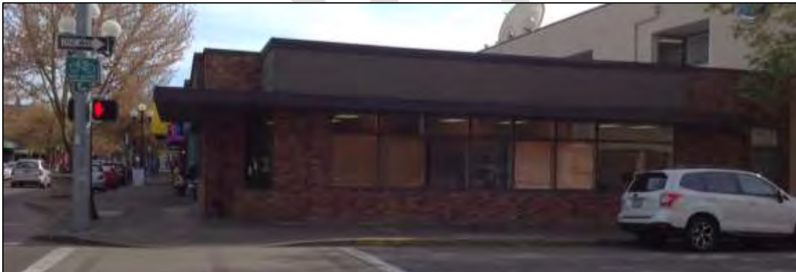
Photos: View of building on 8 th Avenue.
