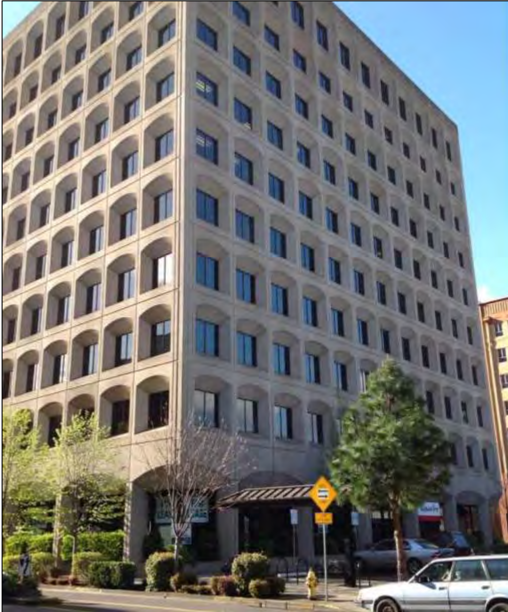
Photos: View of building on Oak Street.
