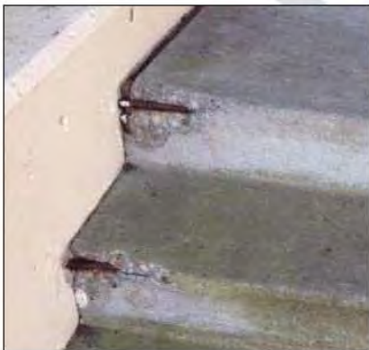
Photo: Top: image of property from Oak Street and East 6 th Avenue; bottom left: image shows rebar in deteriorated stairs; bottom middle: cracks shown on stairwell; bottom right: image shows example of visible repairs.
