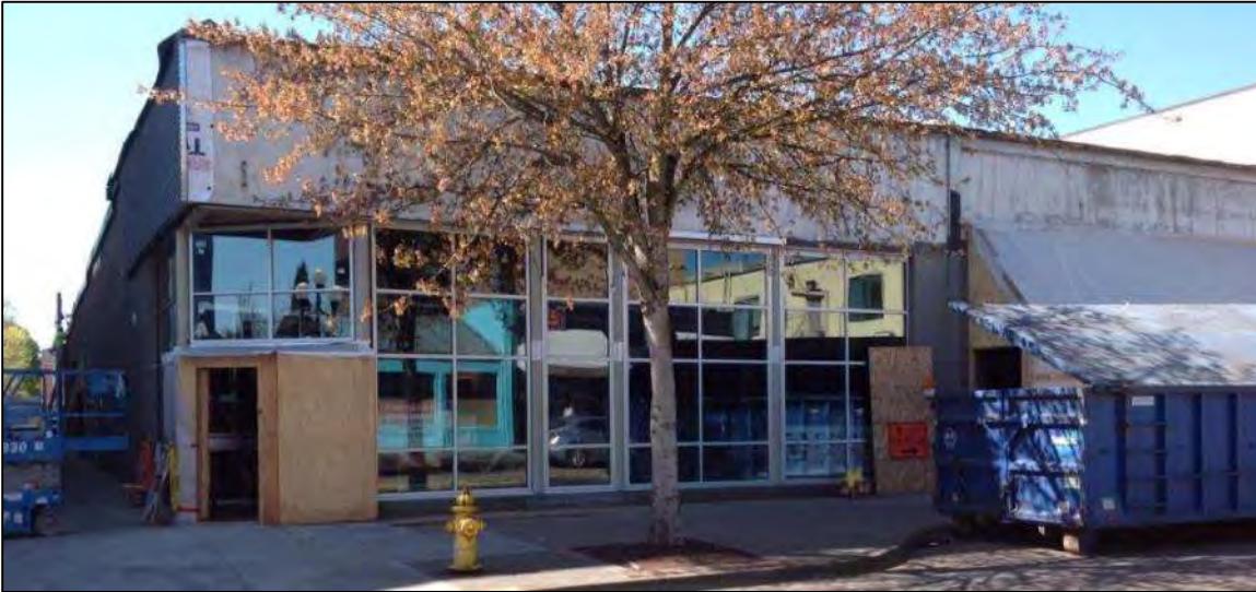
Photo: View of property from Olive Street.
