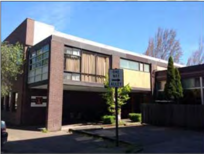
Photo: Top: front of building on Pearl Street; bottom: image shows back of building on Park St.
