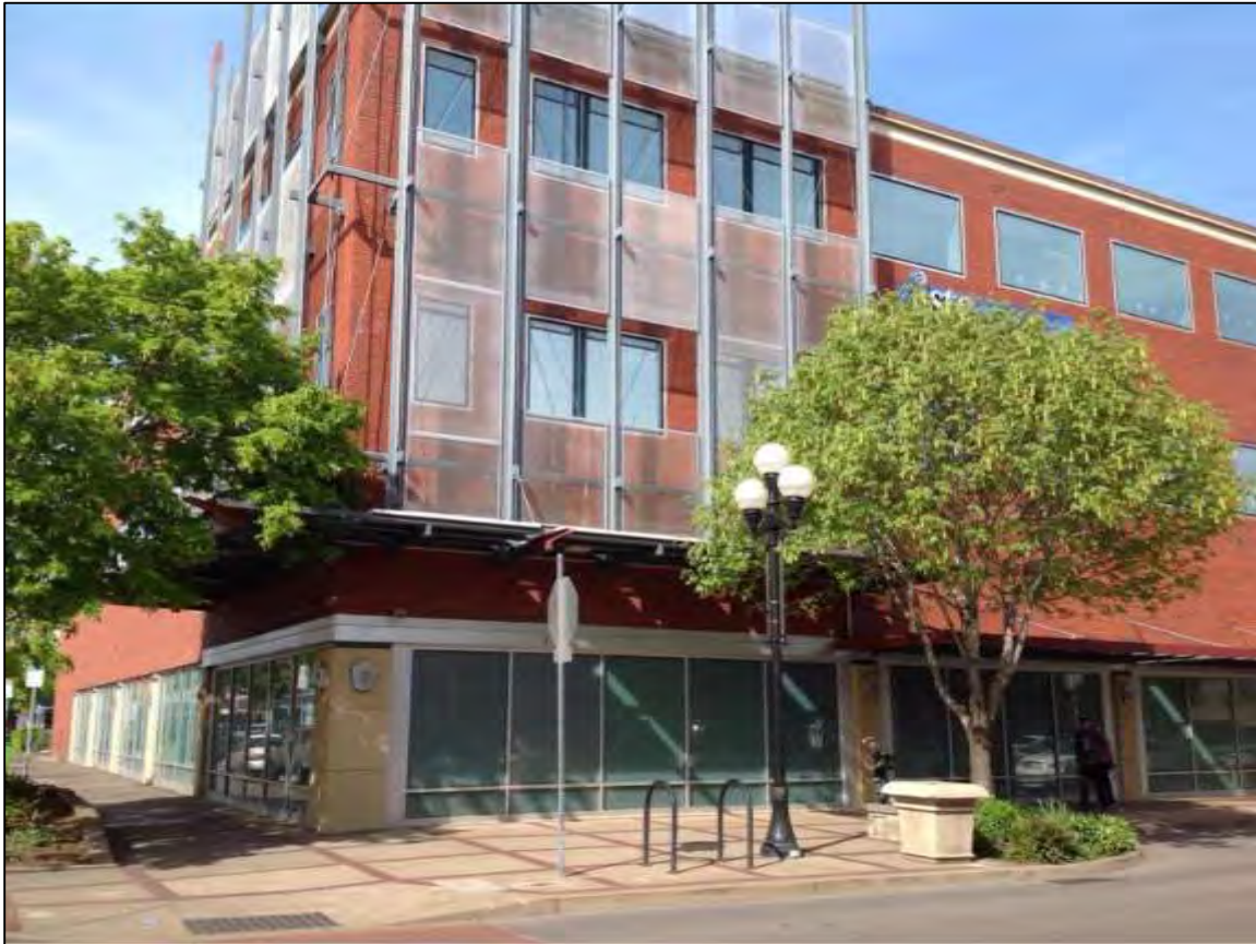
Photo: View of property from Broadway and Charnelton Street.
