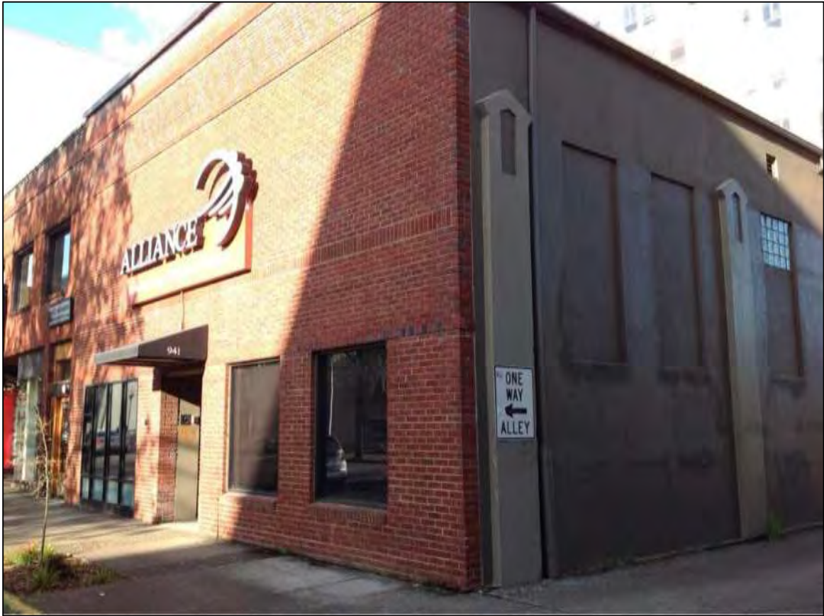
Photos: Building front facing Oak Street.
