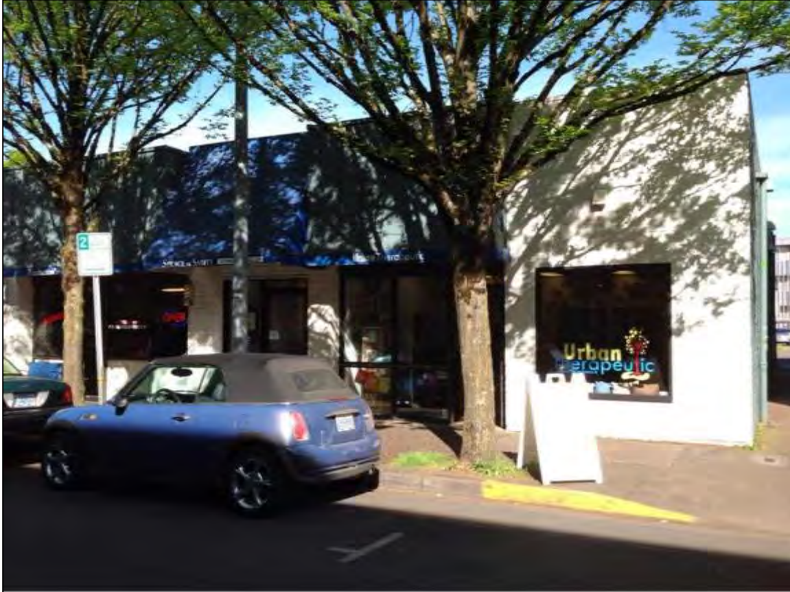
Photos: Front of building facing Willamette Street.
