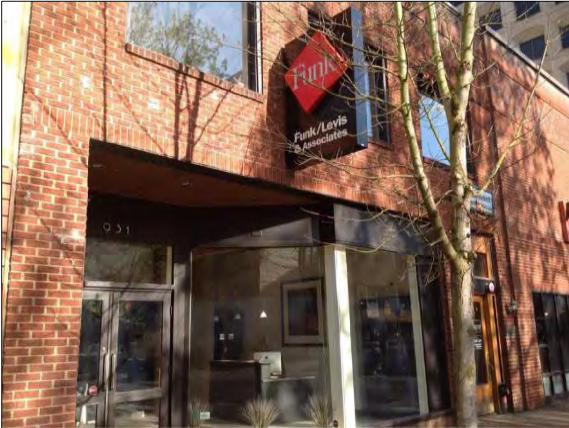
Photo: View of property from Oak Street.
