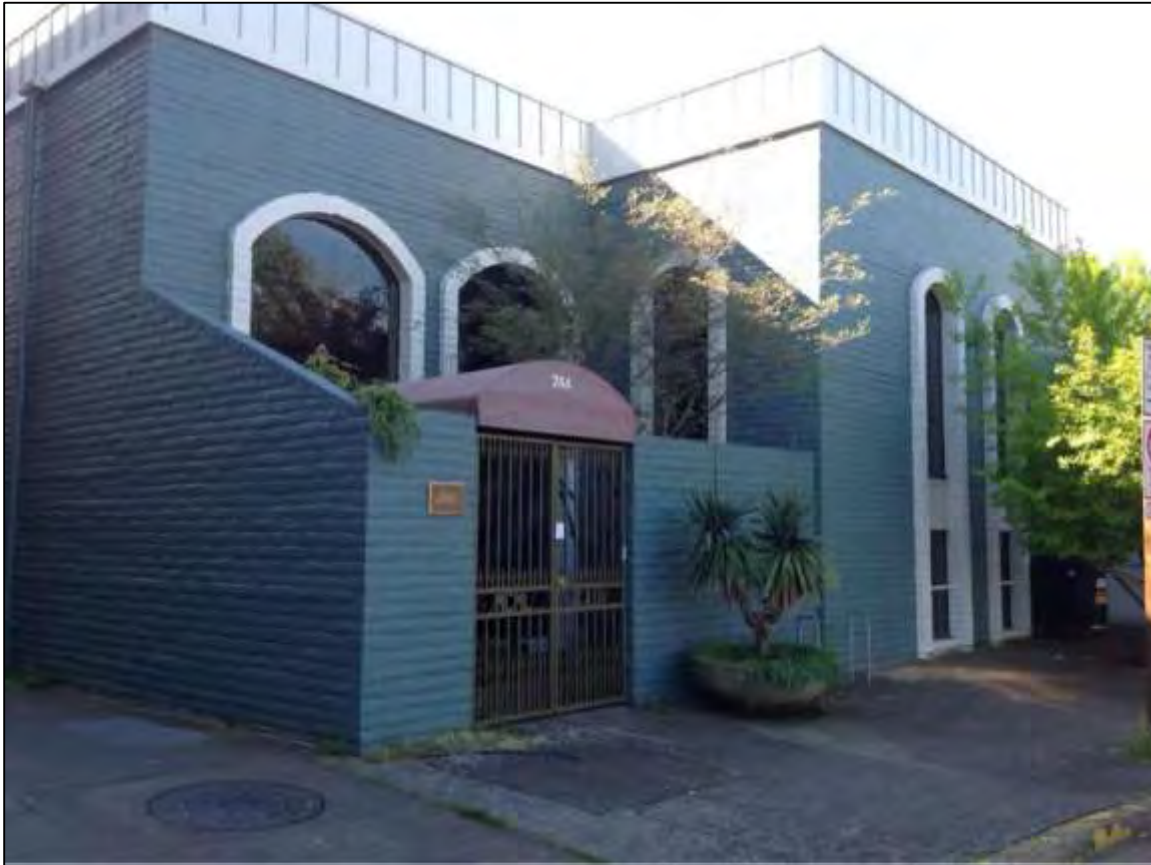
Photos: Building front facing West Park Street.
