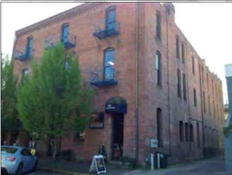
Photo: Top: View of property from Willamette Street, bottom: back of property on West Park Street.
