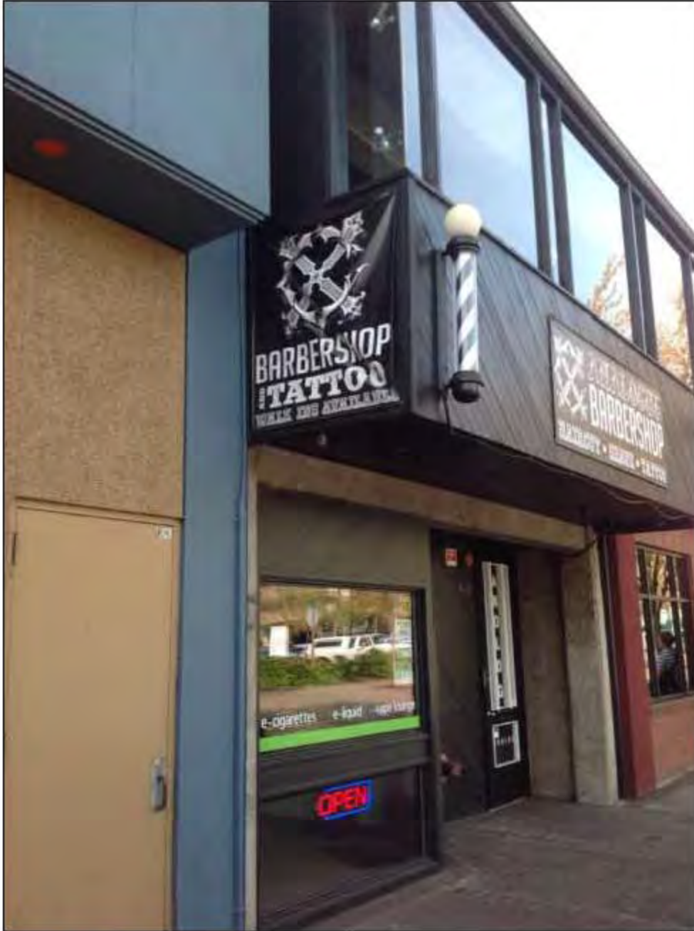
Photos: Front of building facing Olive Street.
