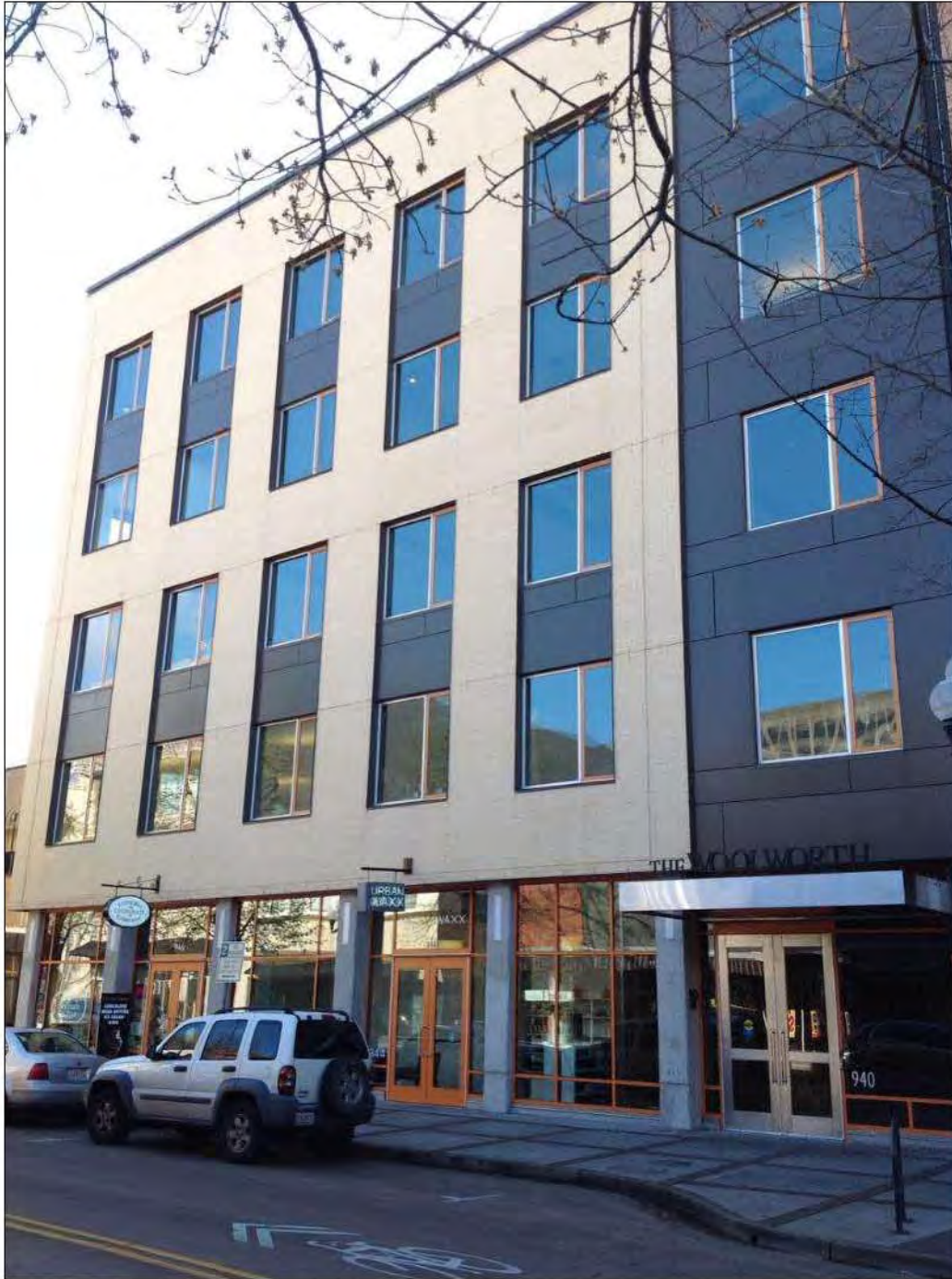
Photo: View of property facing Willamette street.
