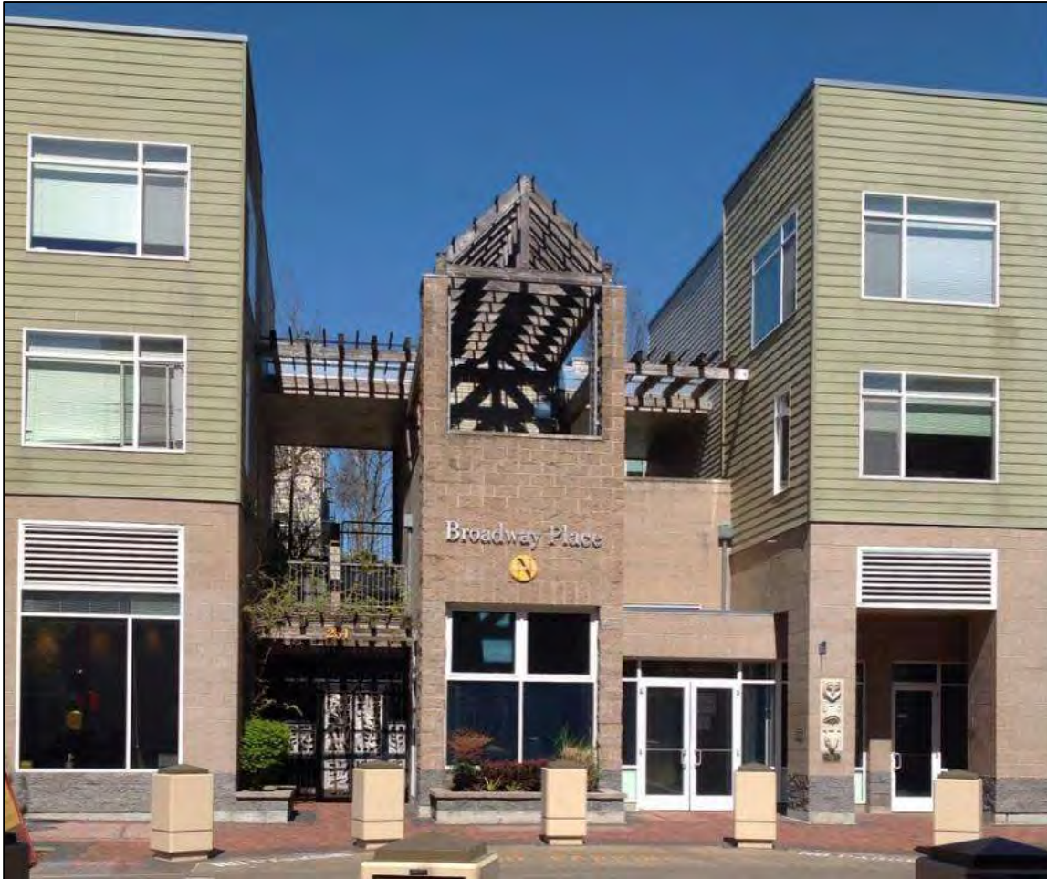
Photos: View of property mid-block on Broadway.
