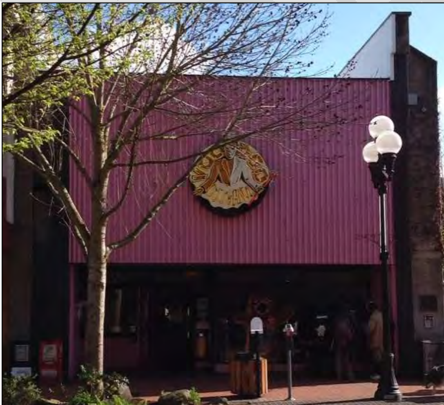
Photo: View of building front from Broadway.
