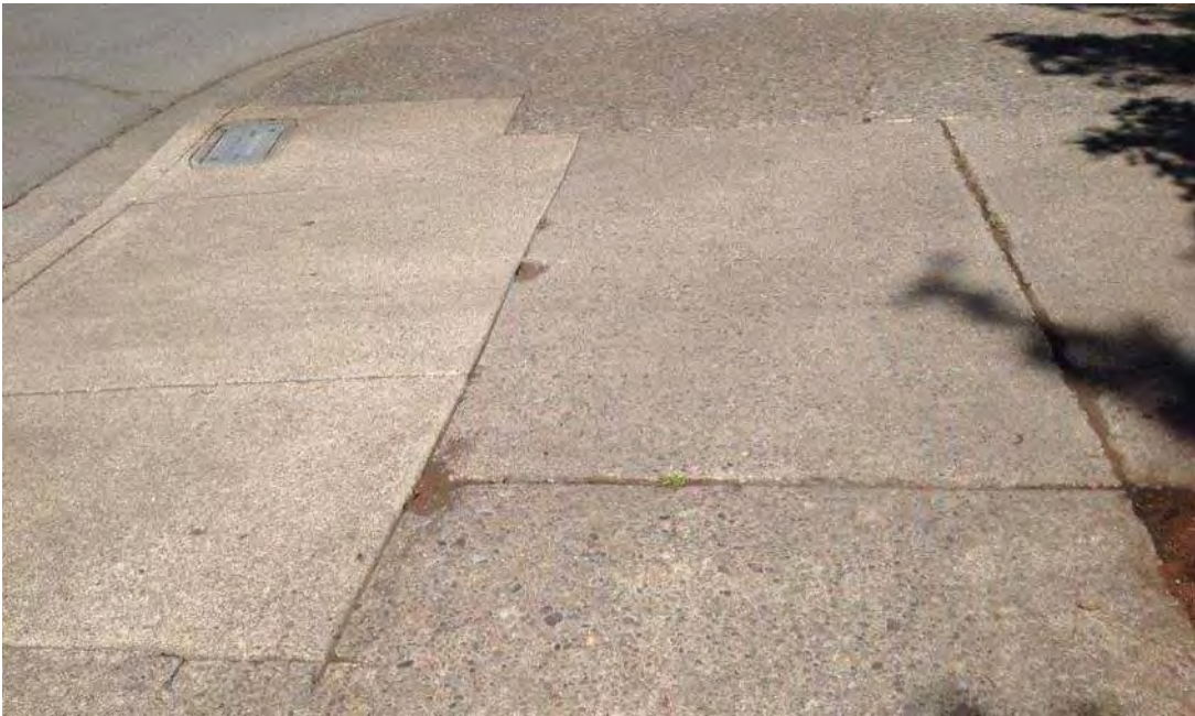
Photo: Top: view of property from Oak Street; bottom: image shows holes and cracks in pavement leading up to ramp
