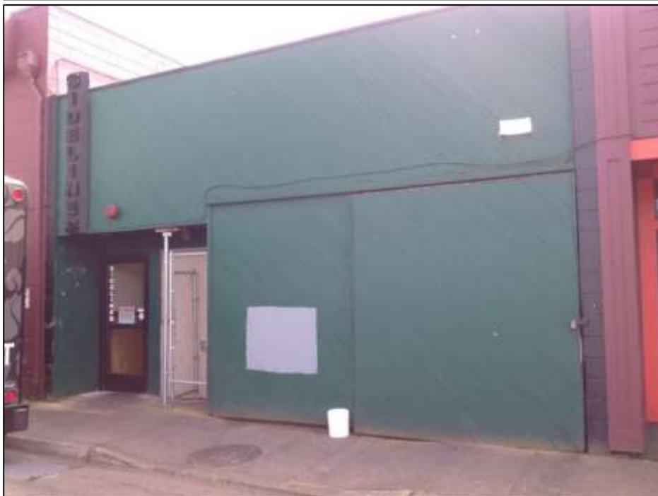
Photo: Top: front of property facing Broadway; bottom: rear of building.
