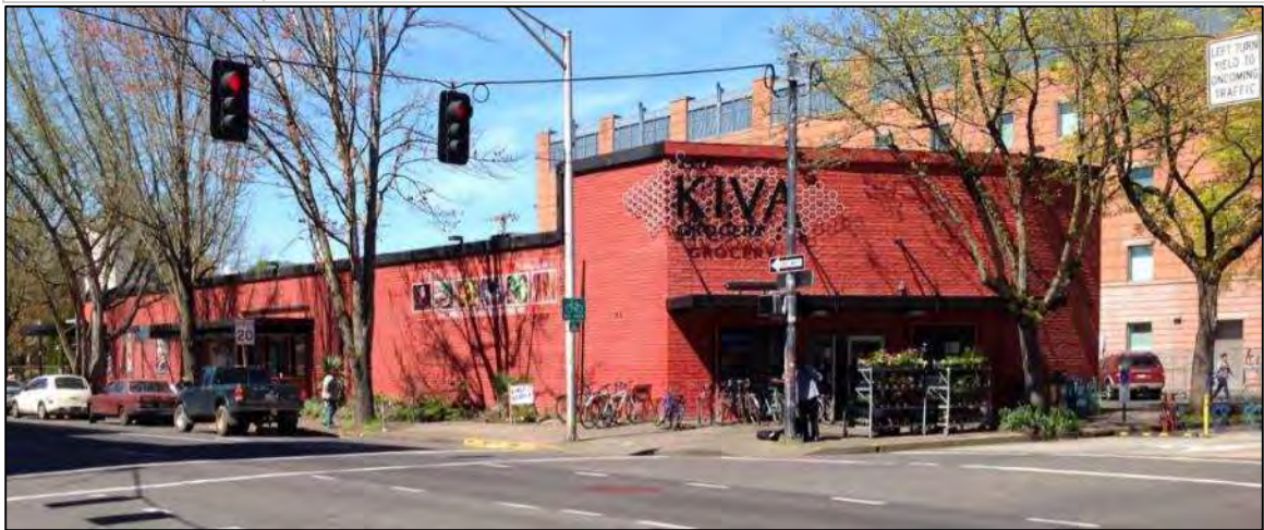
Photo: View of property from 11 th Avenue and Olive Street.
