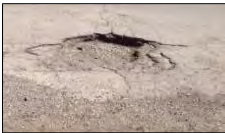
Photos: Top: front of building facing Broadway and Willamette Street; middle left: damage on building ground line; middle right: exposed pipes on building ground line; bottom: damage on parking lot.
