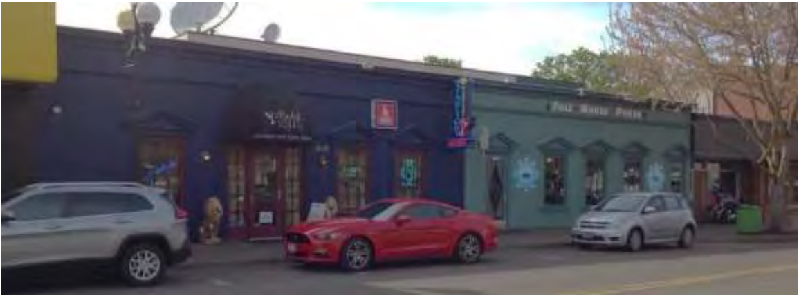
Photo: View of property on Olive Street.
