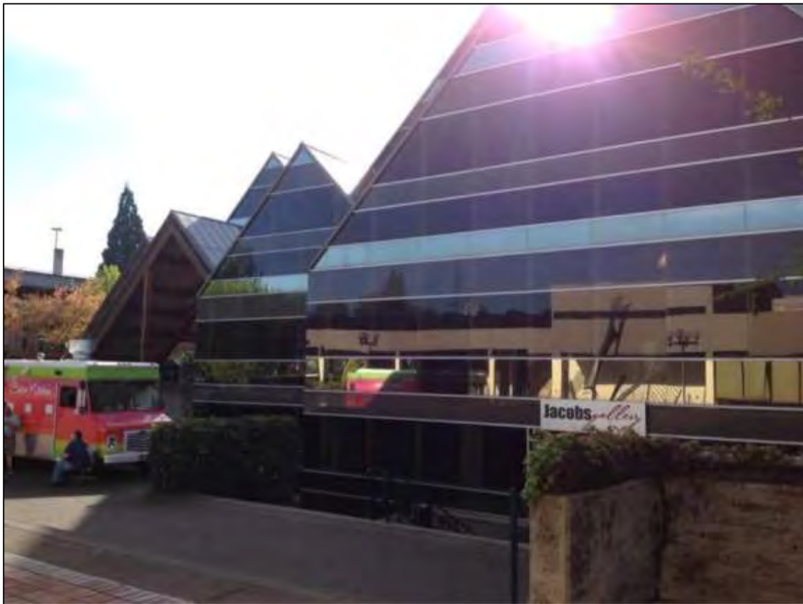
Photo: View of building from pedestrian pathway between conference center and Hult Center.
