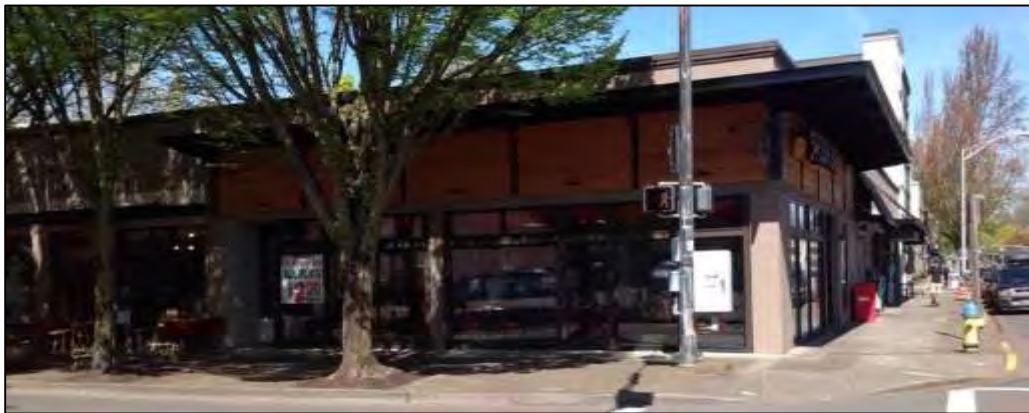
Photos: Top: view of property along East Broadway; bottom: view of building from East Broadway and Pearl Street.
