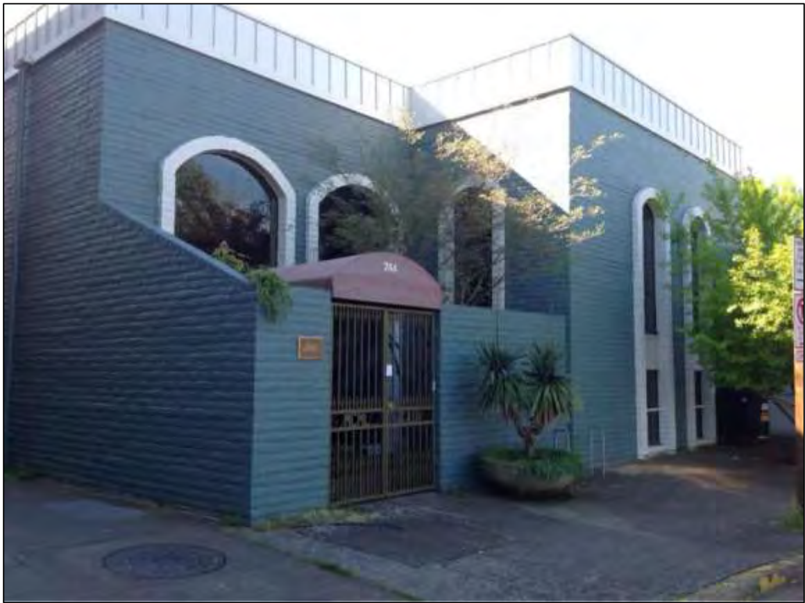
Photos: Building front facing West Park Street.
