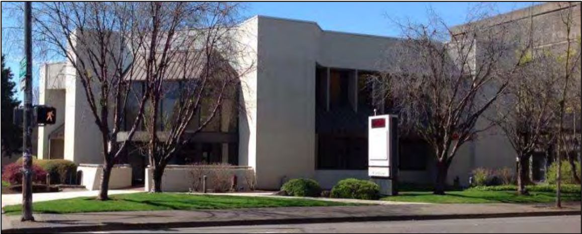
Photo: View of property from East 11 th Avenue and Oak Street.
