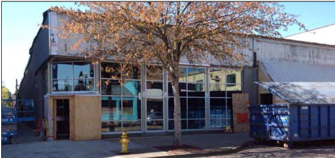
Photo: View of property from Olive Street.
