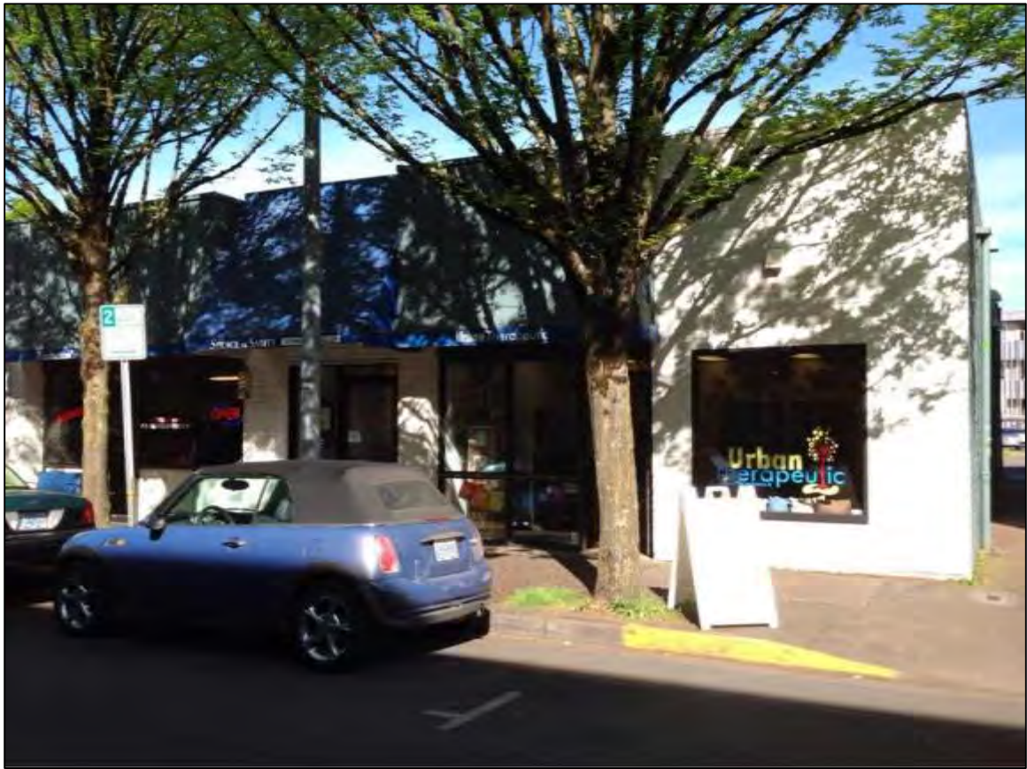
Photos: Front of building facing Willamette Street.
