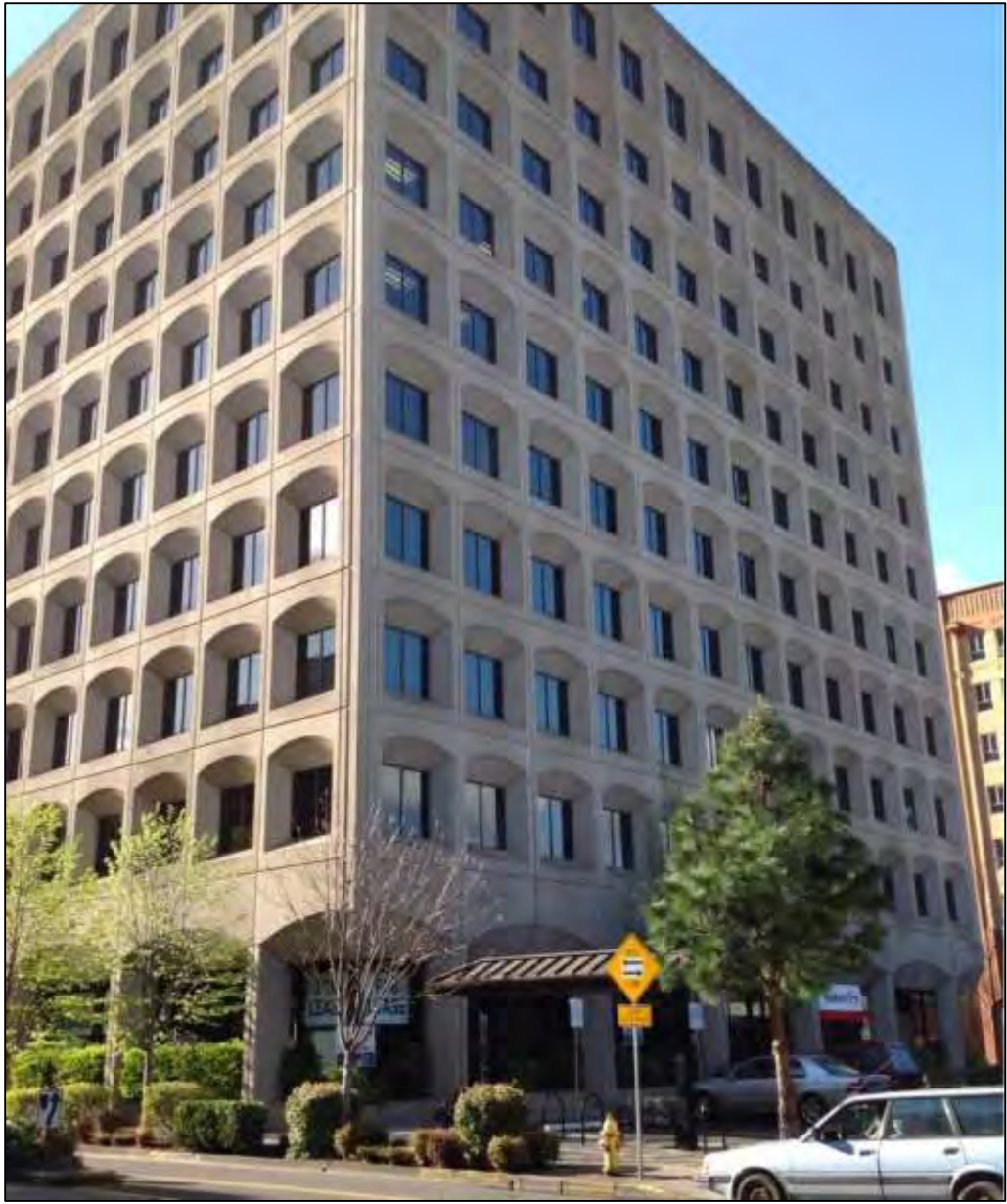
Photos: View of building on Oak Street.
