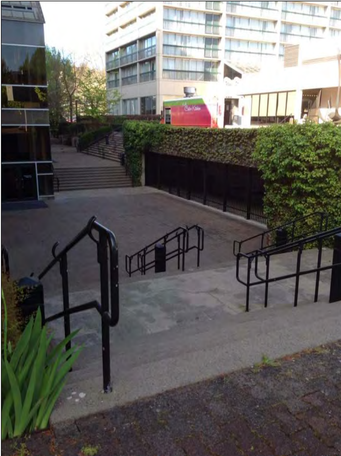
Photo: Image shows open space area, cracks in pavement in stairs landing, and bricks used to create pathways.
