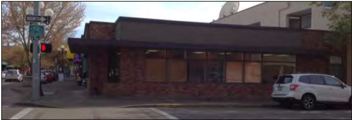
Photos: View of building on 8 th Avenue.
