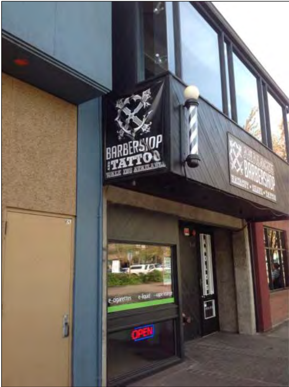
Photos: Front of building facing Olive Street.
