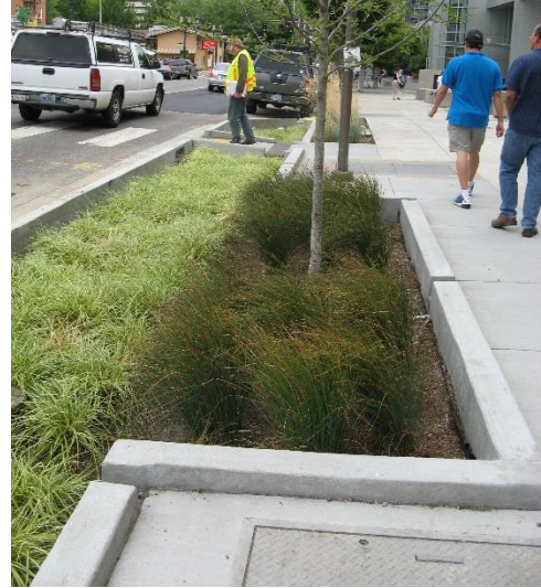
Stormwater treatment can be an attractive part of the streetscape.
