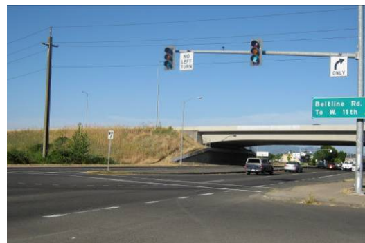
Barger Drive at Randy Papé Bellline is a minor arterial with a curb to curb width of 88 feet.
