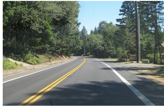
Many roads in Eugene's South Hills lack sidewalks on one or both sides.
