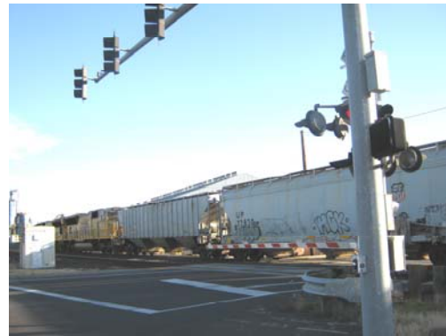
The At-Grade Railroad Crossing at Irvington Drive and NW Expressway.
