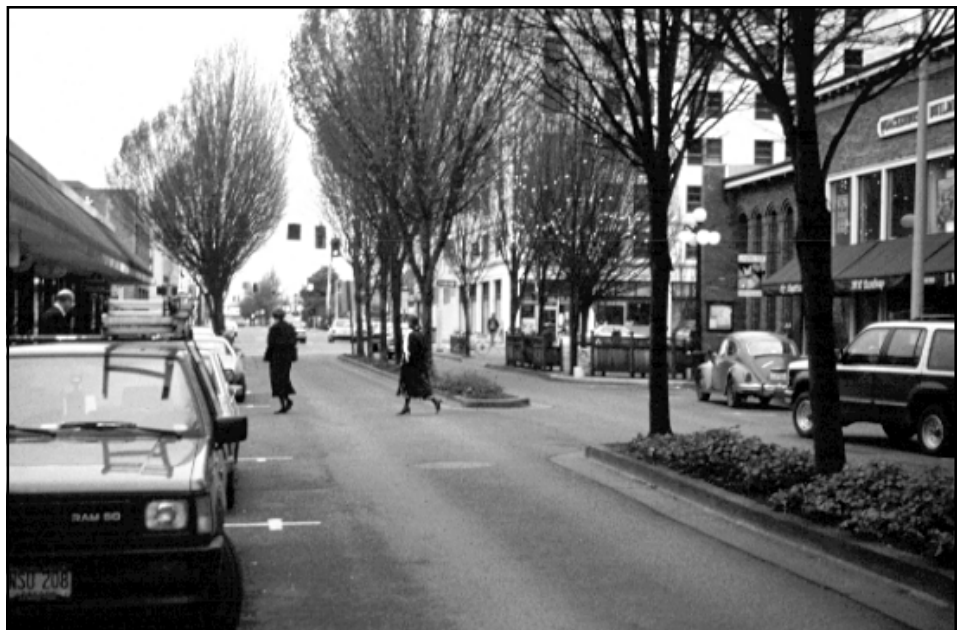
A narrow median, curb extensions, and recessed parking calm traffic on E. Broadway, a downtown collector street
