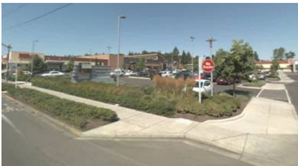
Woodfield Station on 29 th Avenue, west of Willamette Street.
