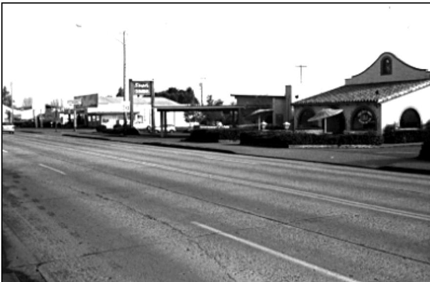
Areas with multiple curb cuts increase accident potential and reduce the efficiency of the street
