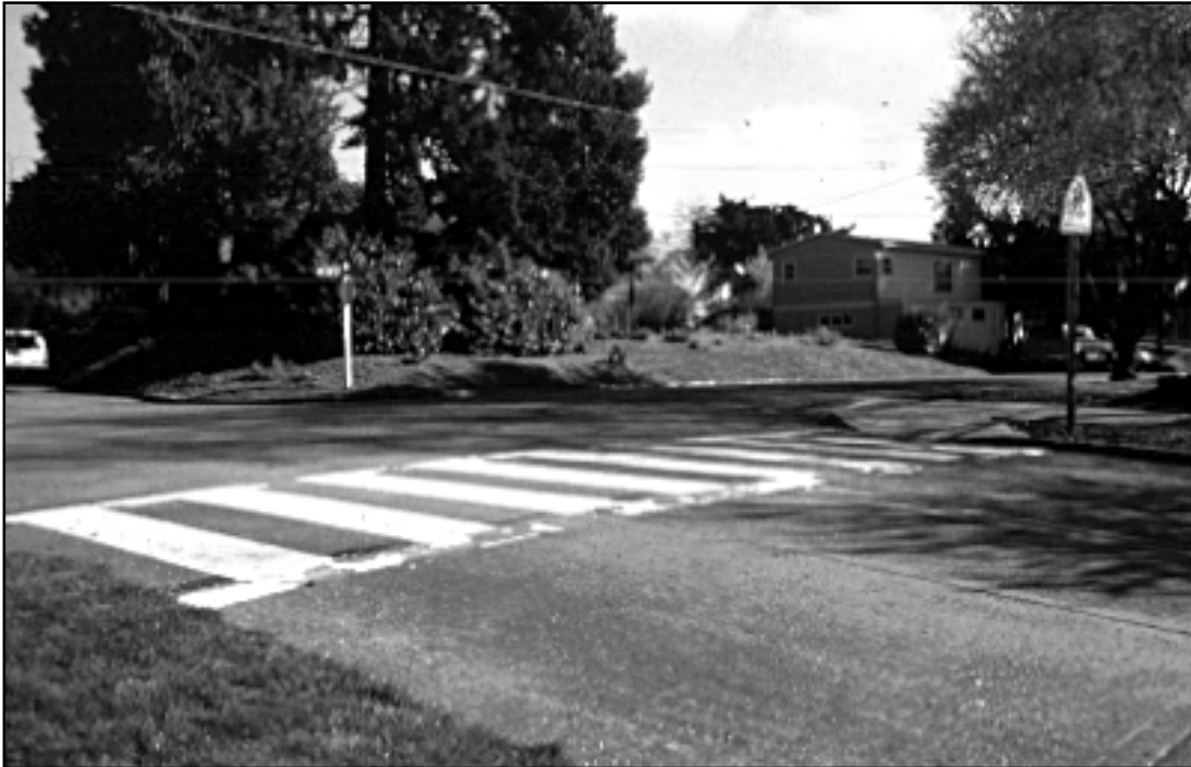
Ladder-style markings increase driver awareness of pedestrian crossing areas
