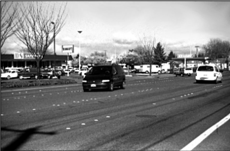
A center turn lane on River Road
