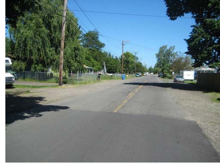
Unimproved roadways throughout Eugene lack bicycle or pedestrian facilities.
