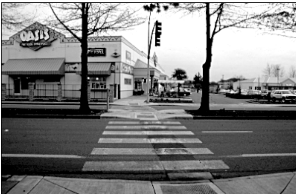
This mid-block crossing improves pedestrian safety on Willakenzie Road near Sheldon High School
