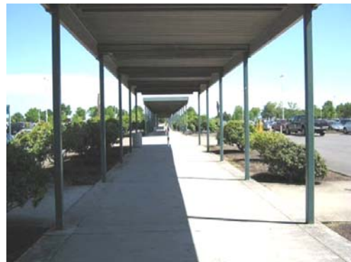
Walkway connecting terminal to parking lot.
