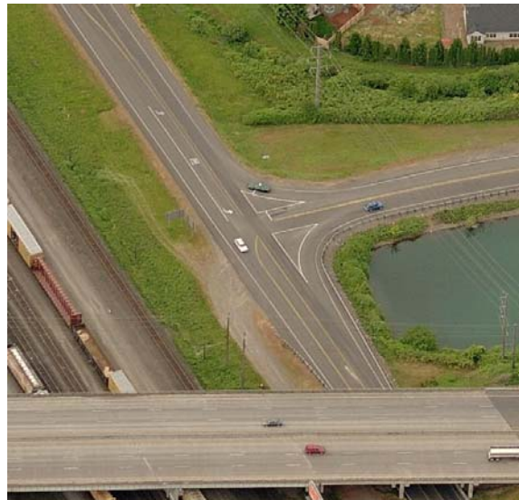
Aerial view of the Randy Papé Beltline Westbound Ramp intersection with Northwest Expressway.
