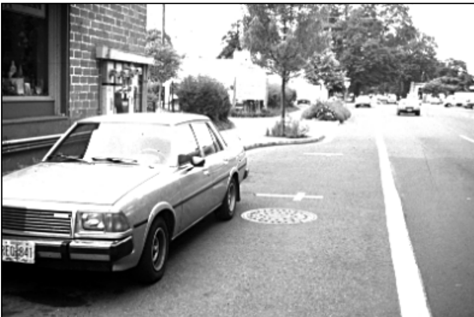
Parking bays, like this one on 5 th Avenue, allow on-street parking while reducing overall street width
