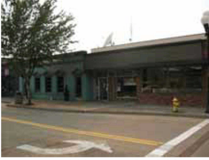
Map ID# 112 —Tax lot 3900 of Map 17033113 (Shoe Repair business/Full House Poker/Former Police Auditor): Single-story building in good shape. Vacancy on corner of Olive and 8 th . Improvement to land ratio: 2.57; Building rating: +
