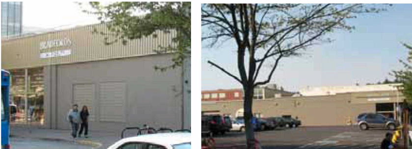
Map ID# 62 —Tax lot 5000 of Map 17033113 (Bradford’s store): Single-story building in good condition. West portion of store is vacant (approximately one-third of structure). EWEB notes that steam conversion is needed. Improvement to land ratio: 1.18; Building rating: +
