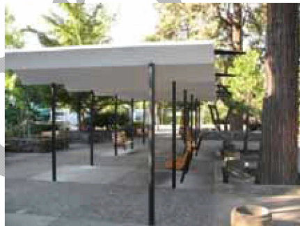
Map ID# 121 —Tax lot 4700 of Map 17033114 (Park Blocks- South): Structures evidence cracking and paint peeling from canopy covering. Improved public plaza. Building rating: ±
