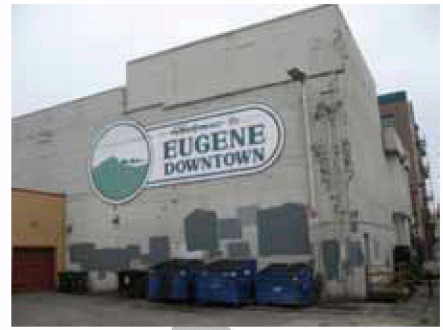
Map ID# 92 —Tax lot 1100 of Map 17033113 (Taco Time Building): Cracking, staining from downspouts, torn awning. Vacancy on corner of Broadway and Willamette. Graffiti on back of building. Improvement to land ratio: 1.33; Building rating: ±
