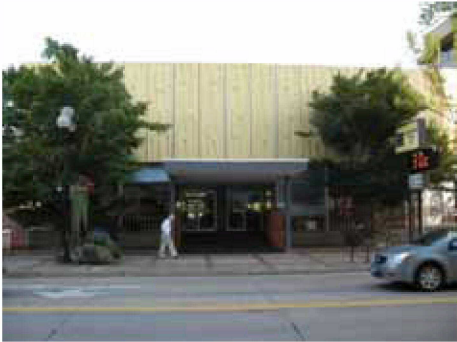
Map ID# 120 —Tax lot 4600 of Map 17033114 (Cascade Title Co.): Building in good condition. Improvement to land ratio: 12.46; Building rating: +
