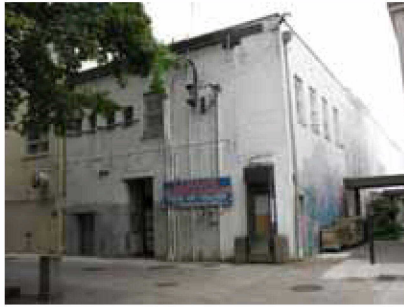
Map ID# 48 —Tax lot 5500 of Map 17033114 (Shoe-a-Holic): Building evidences water damage on exterior, missing bricks, cracks in marble façade, graffiti, exposed external wiring. Recent upgrades completed to front façade only. EWEB notes that steam conversion is needed. Improvement to land ratio: 2.06; Building rating: ±
