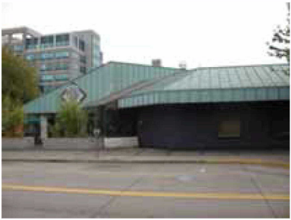
Map ID# 97 —Tax lot 3000 of Map 17033113 (Horsehead Bar): Single-story building. Roof repair and maintenance needed; brick work needs repair. Vacancy along Olive St. Improvement to land ratio: 0.59; Building rating: ±
