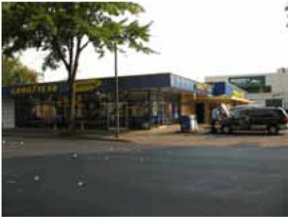
Map ID# 137 —Tax lot 15100 of Map 17033112 (Goodyear Tire): Single-story building in good condition. Improvement to land ratio: .71; Building rating: +
