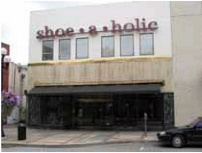
Map ID# 48 —Tax lot 5500 of Map 17033114 (Shoe-a-Holic): Building evidences water damage on exterior, missing bricks, cracks in marble façade, graffiti, exposed external wiring. Recent upgrades completed to front façade only. EWEB notes that steam conversion is needed. Improvement to land ratio: 2.06; Building rating: ±
