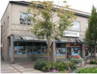
Map ID# 65 —Tax lot 2900 of Map 17033113 (Washburne Building): Building has surface cracking and chipping. Awnings need repairs. One vacancy in building front. EWEB notes that steam conversion is needed. Improvement to land ratio: 3.63; Building rating: ±
