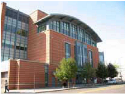
Map ID# 17 —Tax Lot 6500 of Map 17033113 (Eugene Public Library): Library is in good condition and well maintained. Improvement to land ratio: 27.57; Building rating: +
