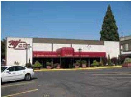
Map ID# 129 —Tax lot 15800 of Map 17033112 (M. Jacobs Furniture): Also associated with Map IDs #141, 142 and 144. Building in good condition. Improvement to land ratio: 1.61; Building rating: +
