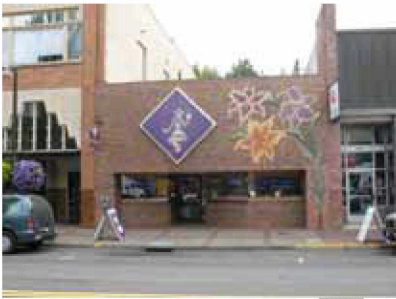
Map ID# 25 —Tax lot 12600 of Map 17033114 (Harlequin Beads): Building appears in good condition. Single-story use. Improvement to land ratio: 2.78; Building rating: +
