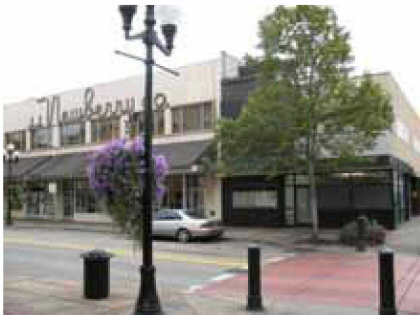
Map ID# 49 —Tax lot 1600 of Map 17033113 (Harry Ritchie's Jewelers): Building appears in good condition. EWEB notes that steam conversion is needed. Improvement to land ratio: 3.85; Building rating: +
