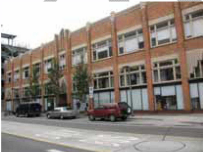
Map ID# 26 —Tax lot 12500 of Map 17033114 (Shaffer Building): Building appears in good condition overall but window frames deteriorating and paint peeling. EWEB notes that steam conversion is needed. Third floor appears vacant. Improvement to land ratio: 9.14; Building rating: ±
