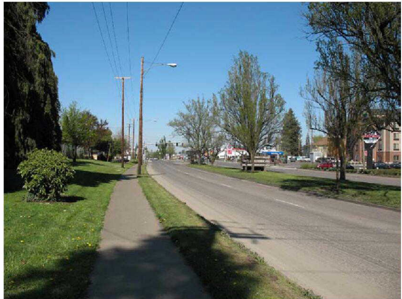
Franklin Boulevard looking east
