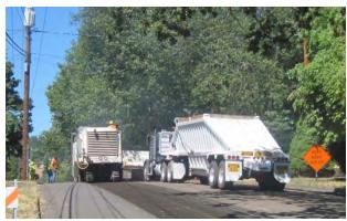
Removing top layers of pavement on 40<sup>th</sup> Avenue for inlay treatment
