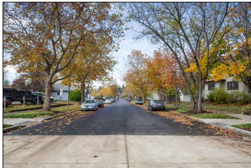
17th Avenue post-project
