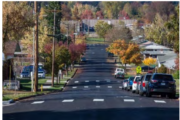
22 nd Avenue post-construction
