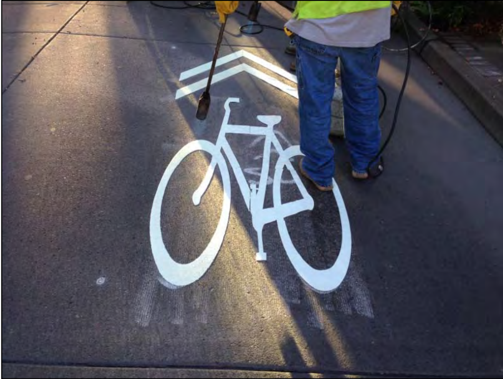
Installation of a shared lane pavement marking in 2015
