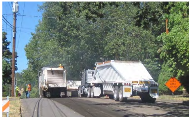
Removing top layers of pavement on 40 th Avenue for inlay treatment
