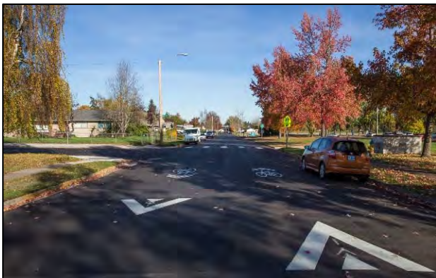
Fillmore Street post-construction
