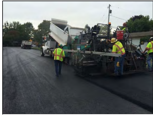
Paving on 19 th Avenue
