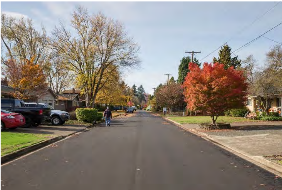
Mahlon Avenue post-construction
