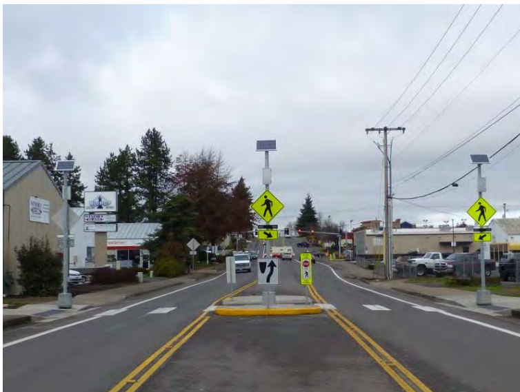
Rectangular rapid flashing beacon crossing installed on Bailey Hill Road
