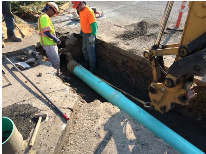
Installation of new stormwater pipe on 22 nd Avenue
