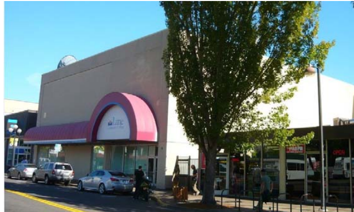
Old LCC Building in its current state
