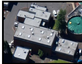
Maintenance Building Aerial
