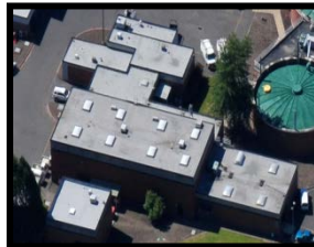
Maintenance Building Aerial
