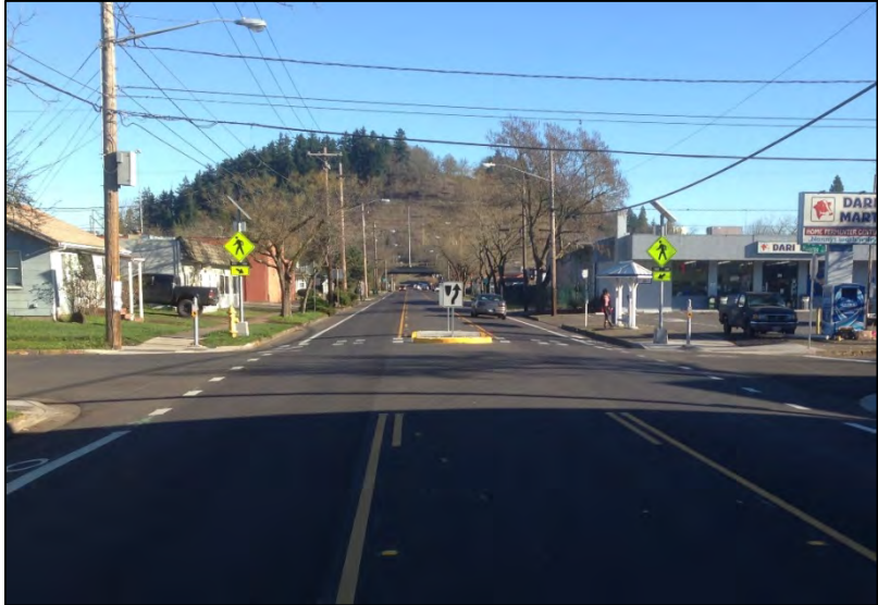
1st Avenue post-project
