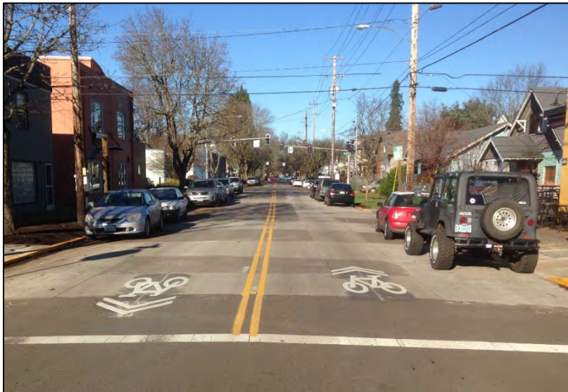
Monroe Street post-project
