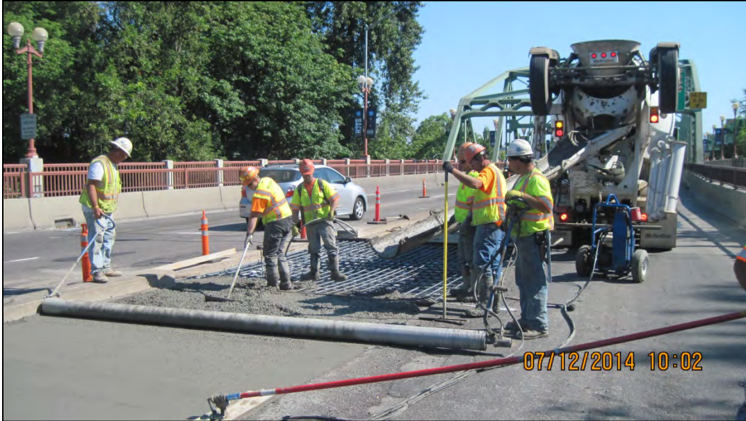
Portland cement concrete overlay paving on Coburg Road between the viaduct and Ferry Street Bridge
