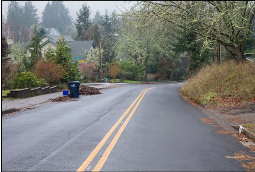
43rd Avenue post-project
