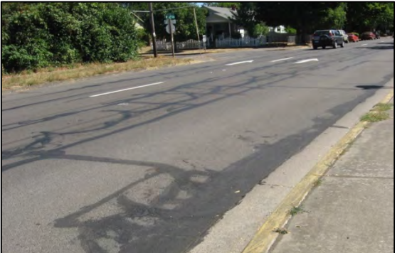
13th Avenue pre-construction
