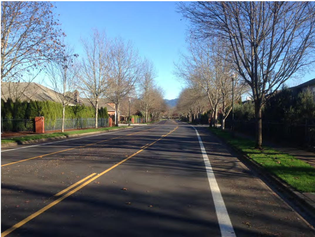
Goodpasture Loop post-construction
