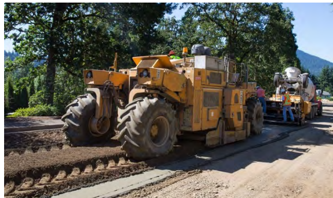
In-place recycling on North Shasta Loop
