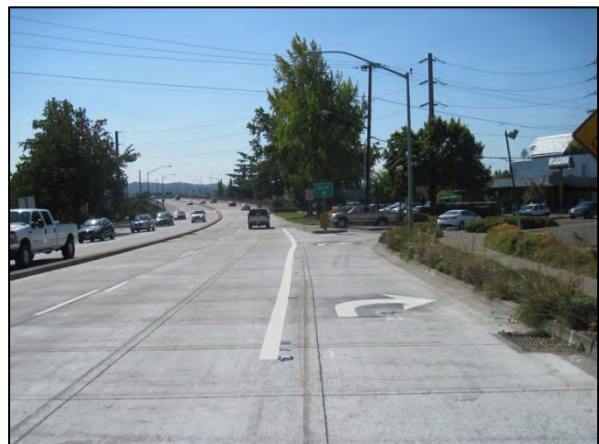
Coburg Road post-construction
