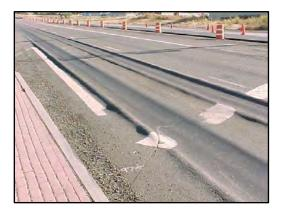
*Joint Spalling:* Spalling is the deterioration of the edges of a concrete slab within 2 feet (0.6m) of the joint. The edges get chipped off concrete slabs causing spalling. Spalling is caused by heavy traffic loads and environmental factors.
