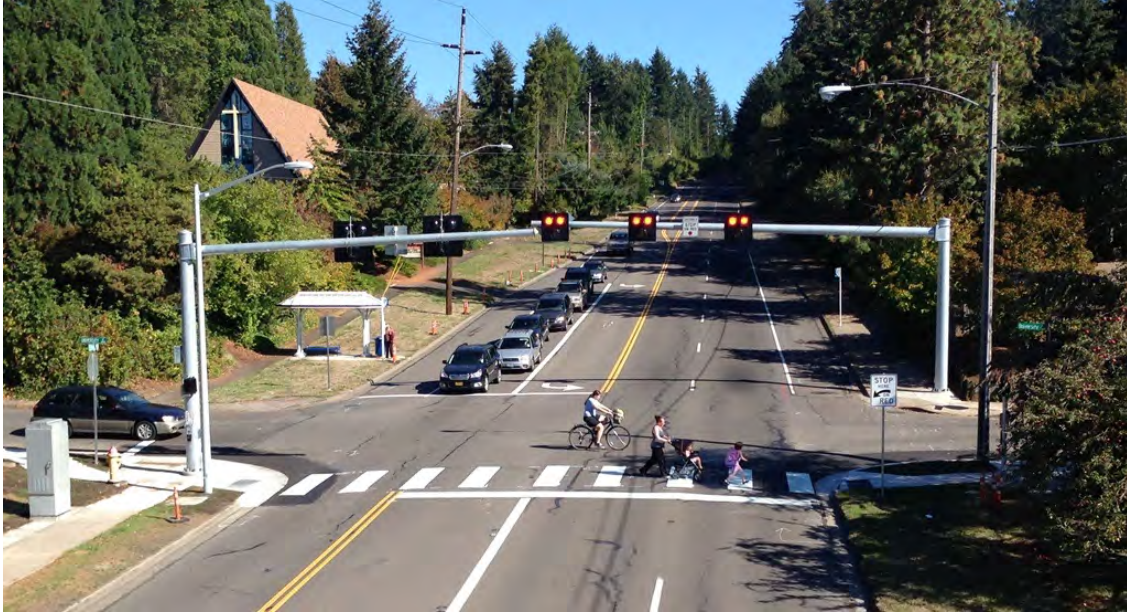
Pedestrian Hybrid Beacon on 30th Avenue
