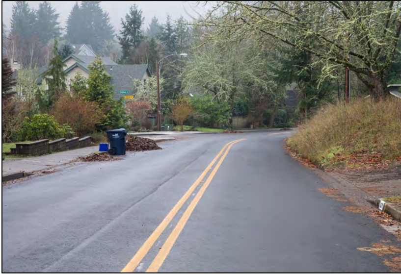
43rd Avenue post-project
