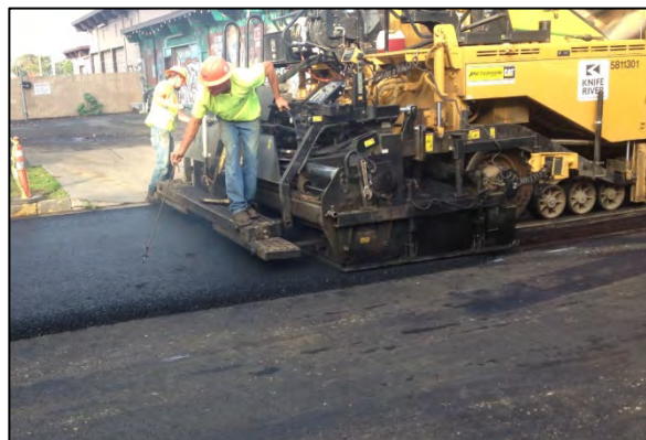
Paving on Monroe Street
