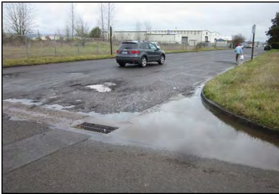
Intersection of 13th and Interior pre-construction
