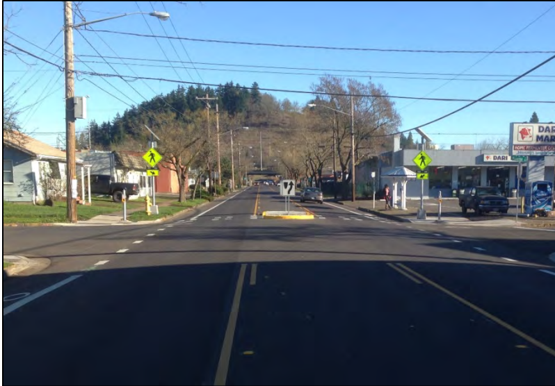
1st Avenue post-project
