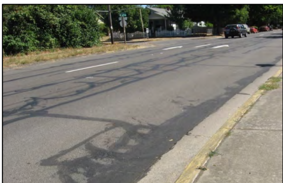
13th Avenue pre-construction
