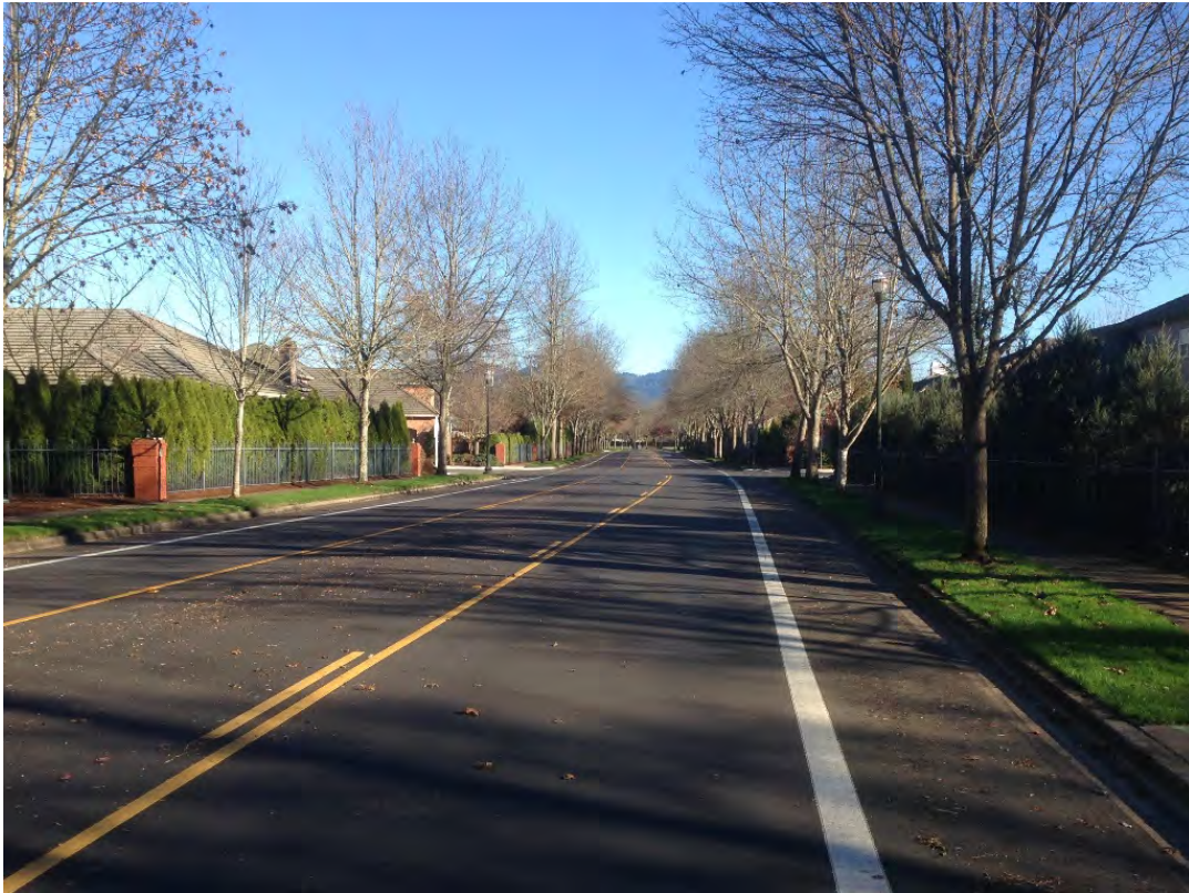
Goodpasture Loop post-construction
