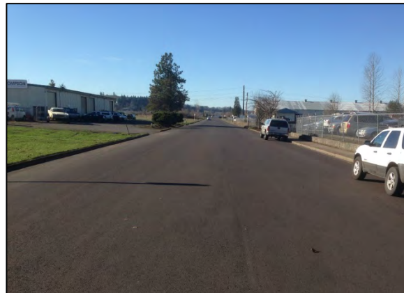
13th Avenue post-construction
