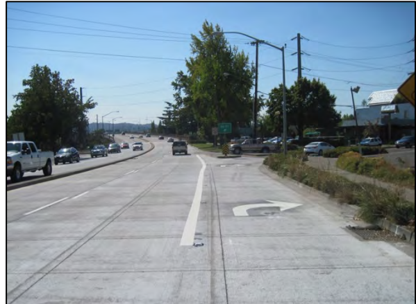
Coburg Road post-construction
