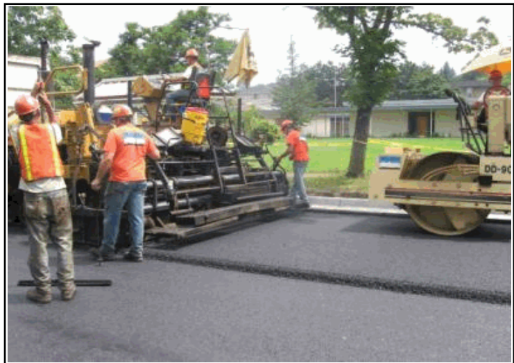
Capital pavement overlay project in progress.
