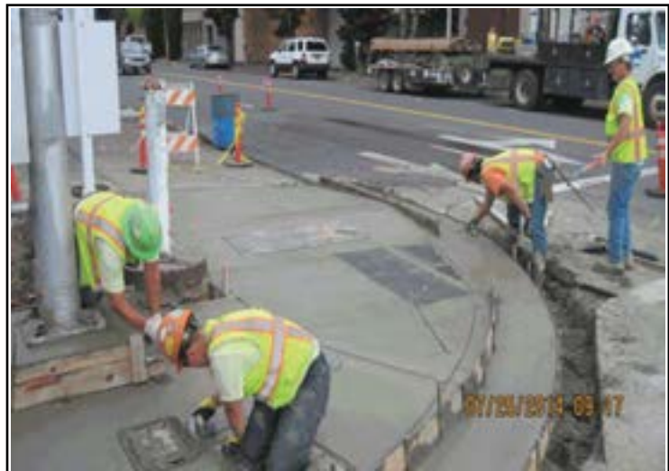
Construction of an accessible sidewalk ramp
