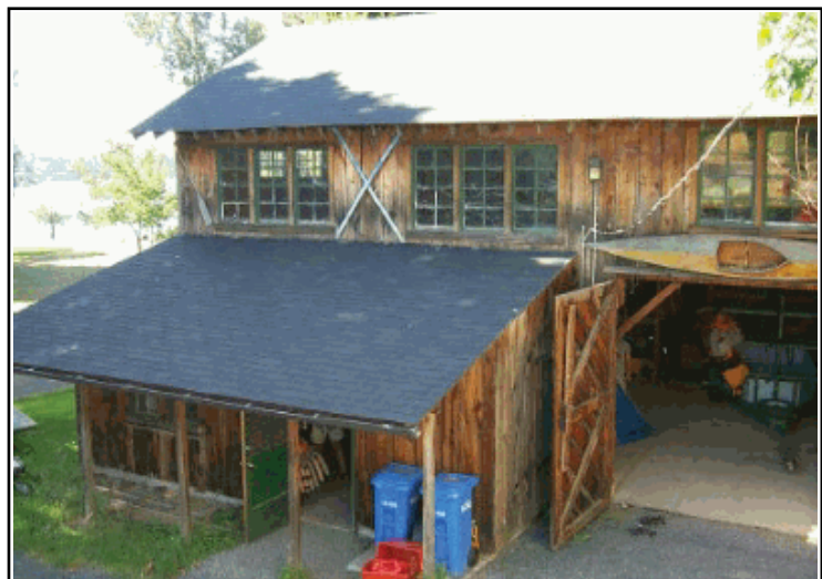
Riverhouse Canoe Storage
