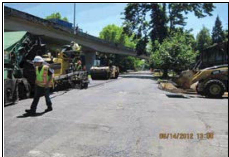
Capital pavement overlay in progress.
