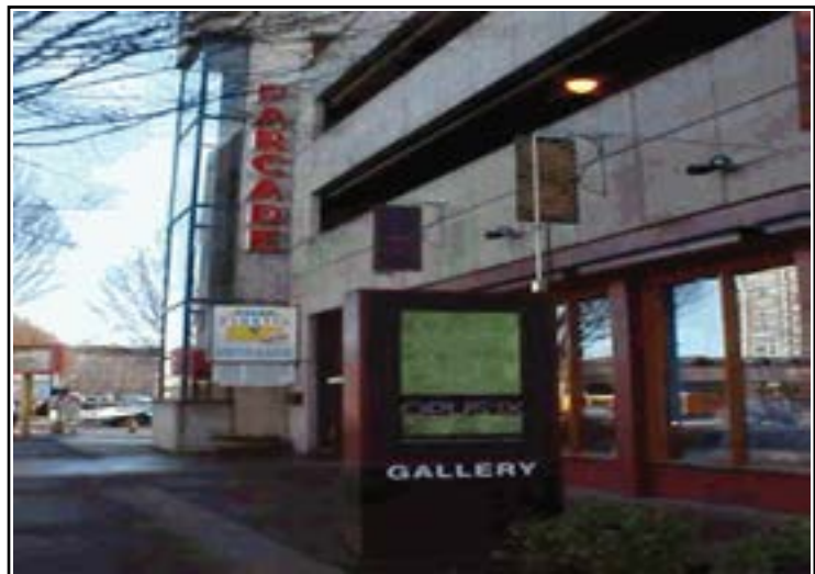
Parcade Parking Garage commercial space
