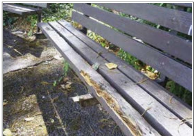
Deteriorating park bench
