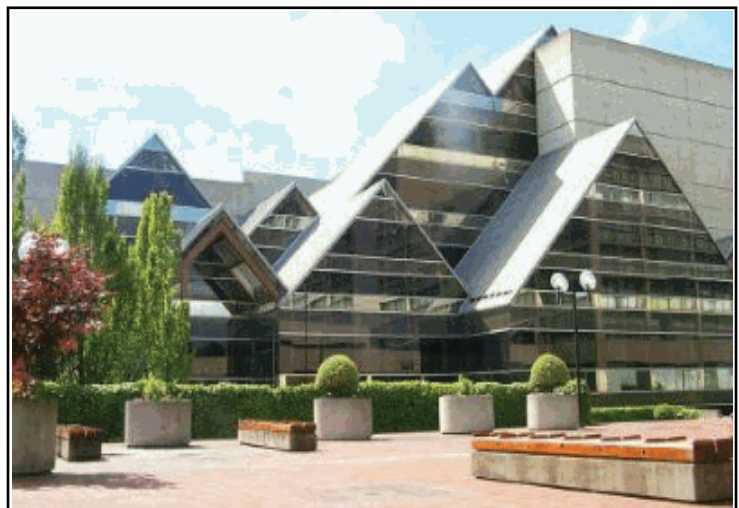
Hult Center is one of the City facilities supported by this project.
