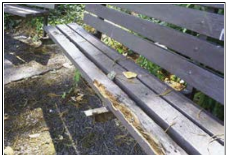
Deteriorating park bench
