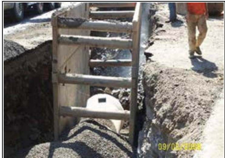
Stormwater line construction underway
