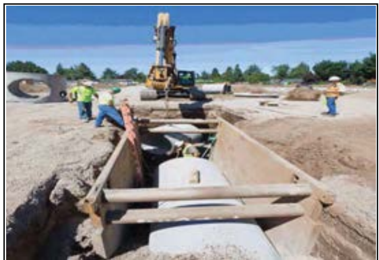
Installing stormwater pipe
