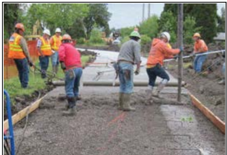
Shared-use path under construction
