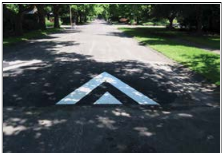
Traffic calming speed hump
