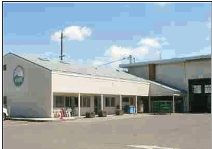
Current Fleet Maintenance facility at 1820 Roosevelt, Eugene.
