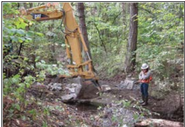
Streambank stabilization work.
