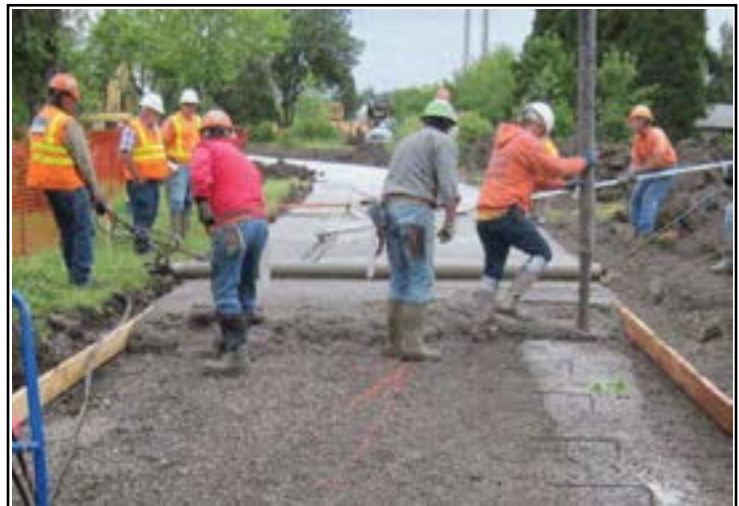
Shared-use path under construction
