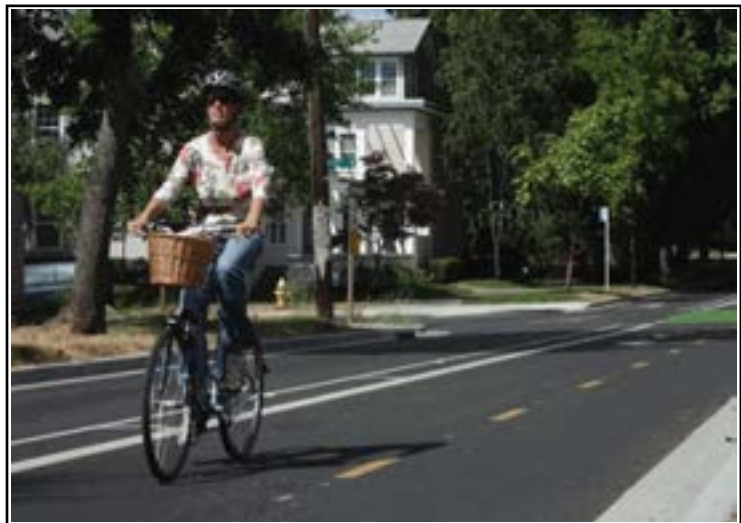
13th Avenue Active Transportation Corridor
