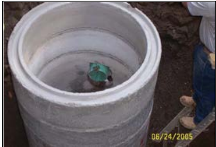
New manholes are one component of the infrastructure that gets built in conjunction with new development.
