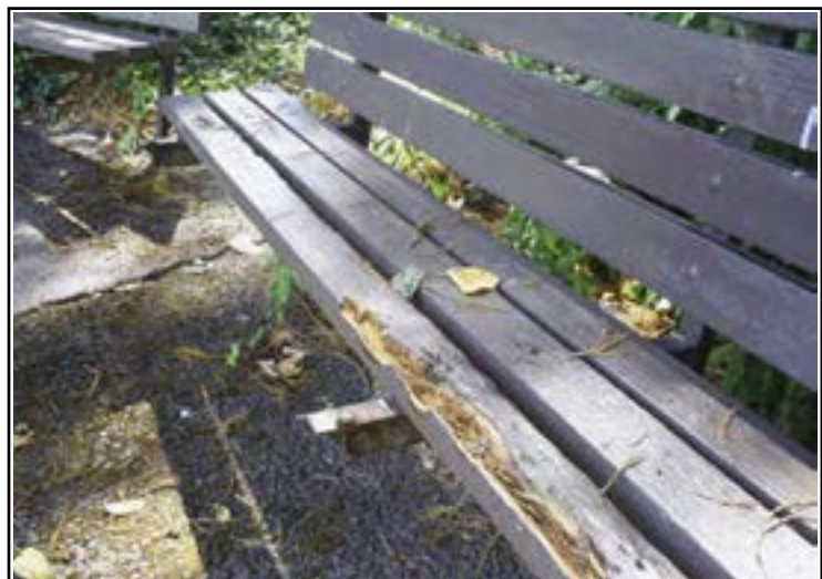
Deteriorating park bench
