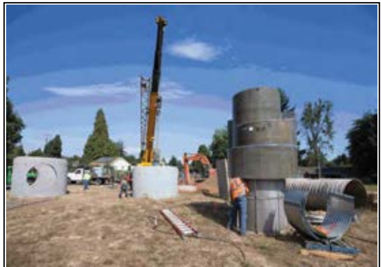
Water Quality Structure
