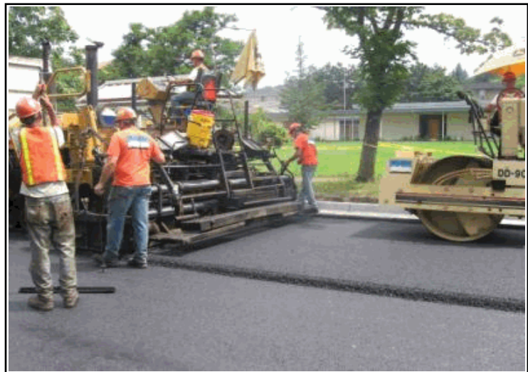
Capital pavement overlay project in progress.
