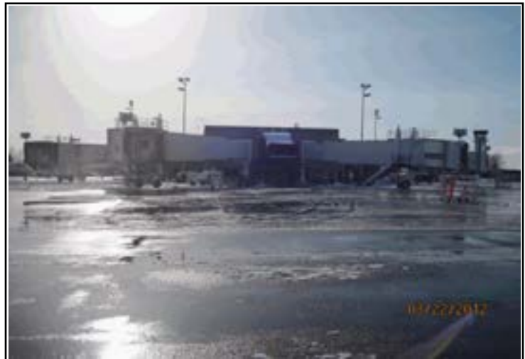
Jet Bridge Replacement
