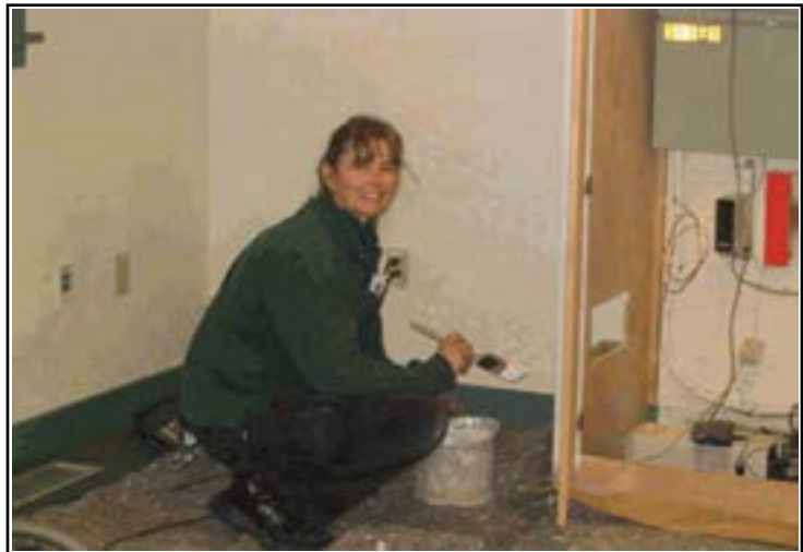
Interior painting at River House.
