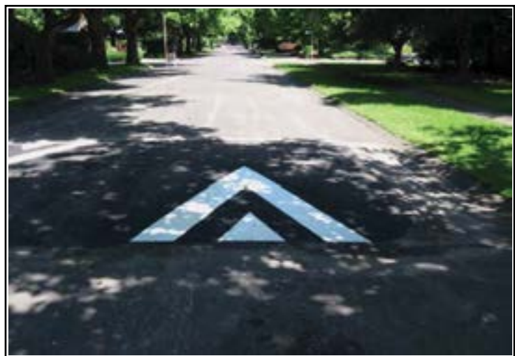
Traffic calming speed hump
