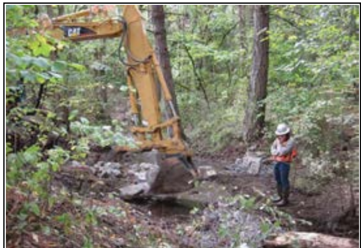
Streambank stabilization work.
