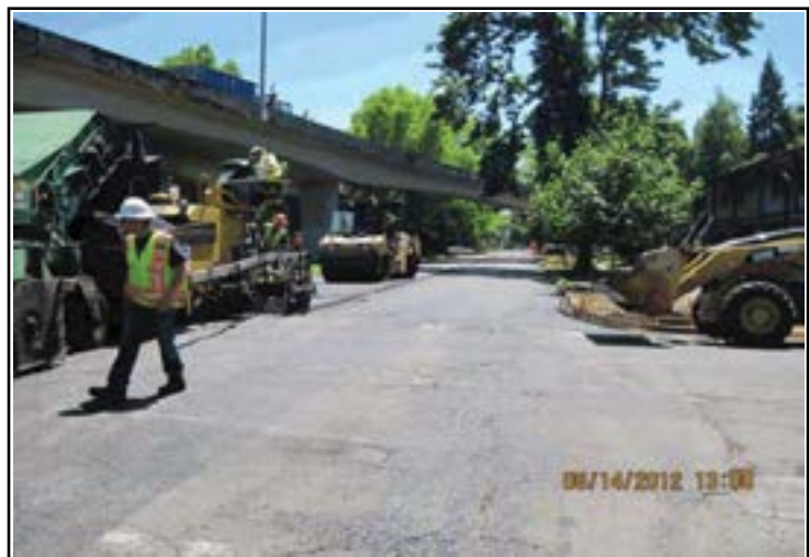
Capital pavement overlay in progress.
