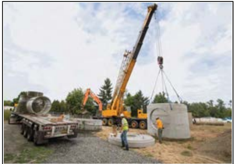
Water Quality Structure
