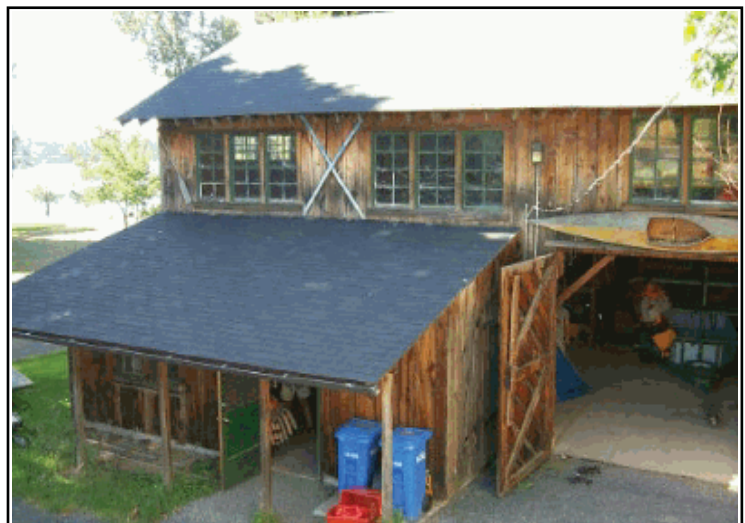
Riverhouse Canoe Storage
