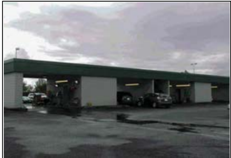
Current Eugene Airport Car Wash Facility
