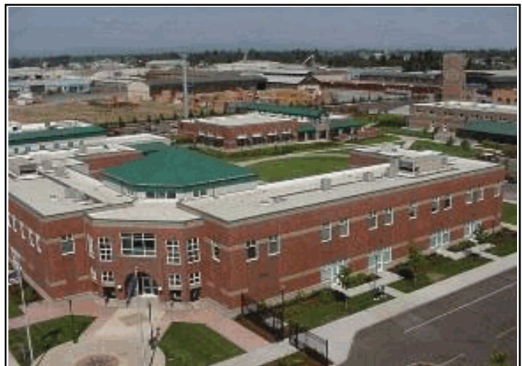
Eugene Fire and EMS headquarters is one of many buildings maintained by the General Fund.
