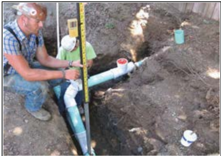
Service line being built at the property line as part of the Community Wastewater Sewers project.
