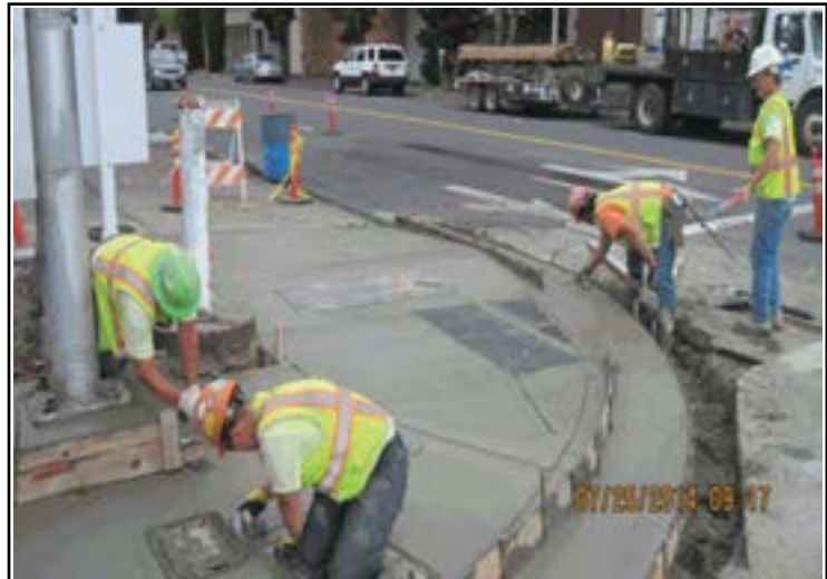
Construction of an accessible sidewalk ramp
