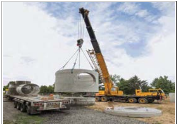
Water Quality Structure
