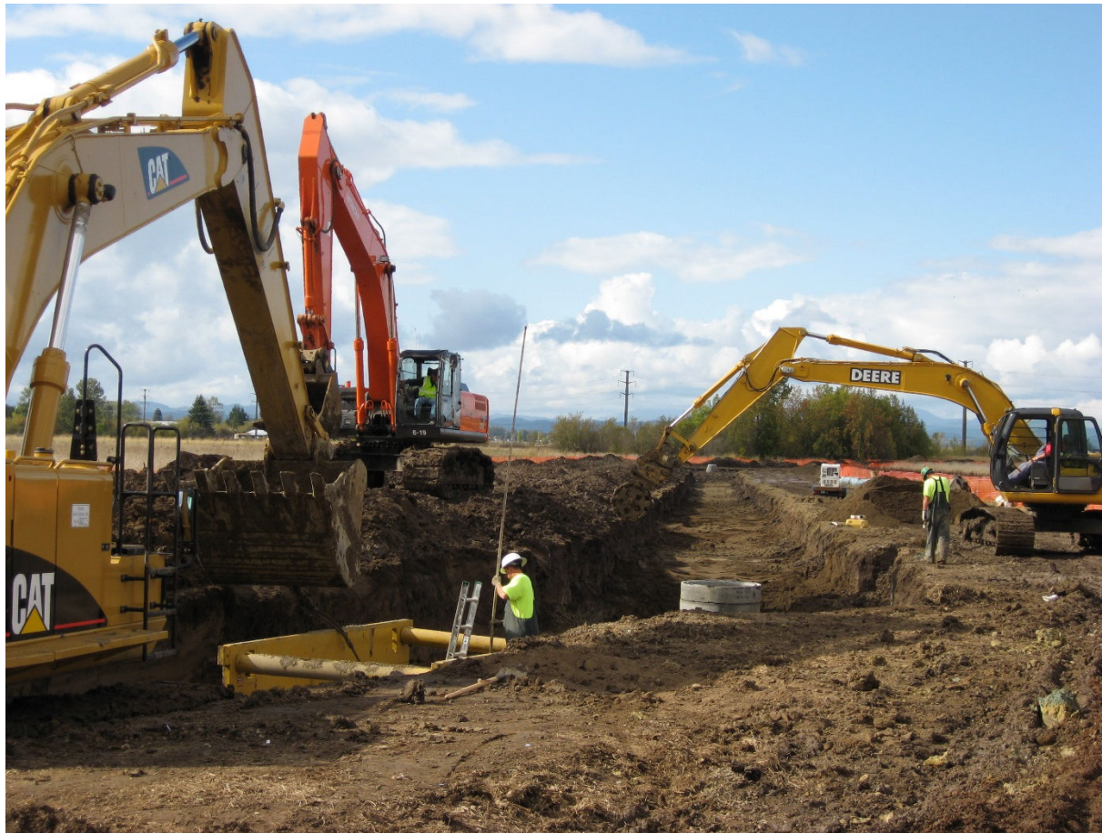
Legacy Wastewater Interceptor
