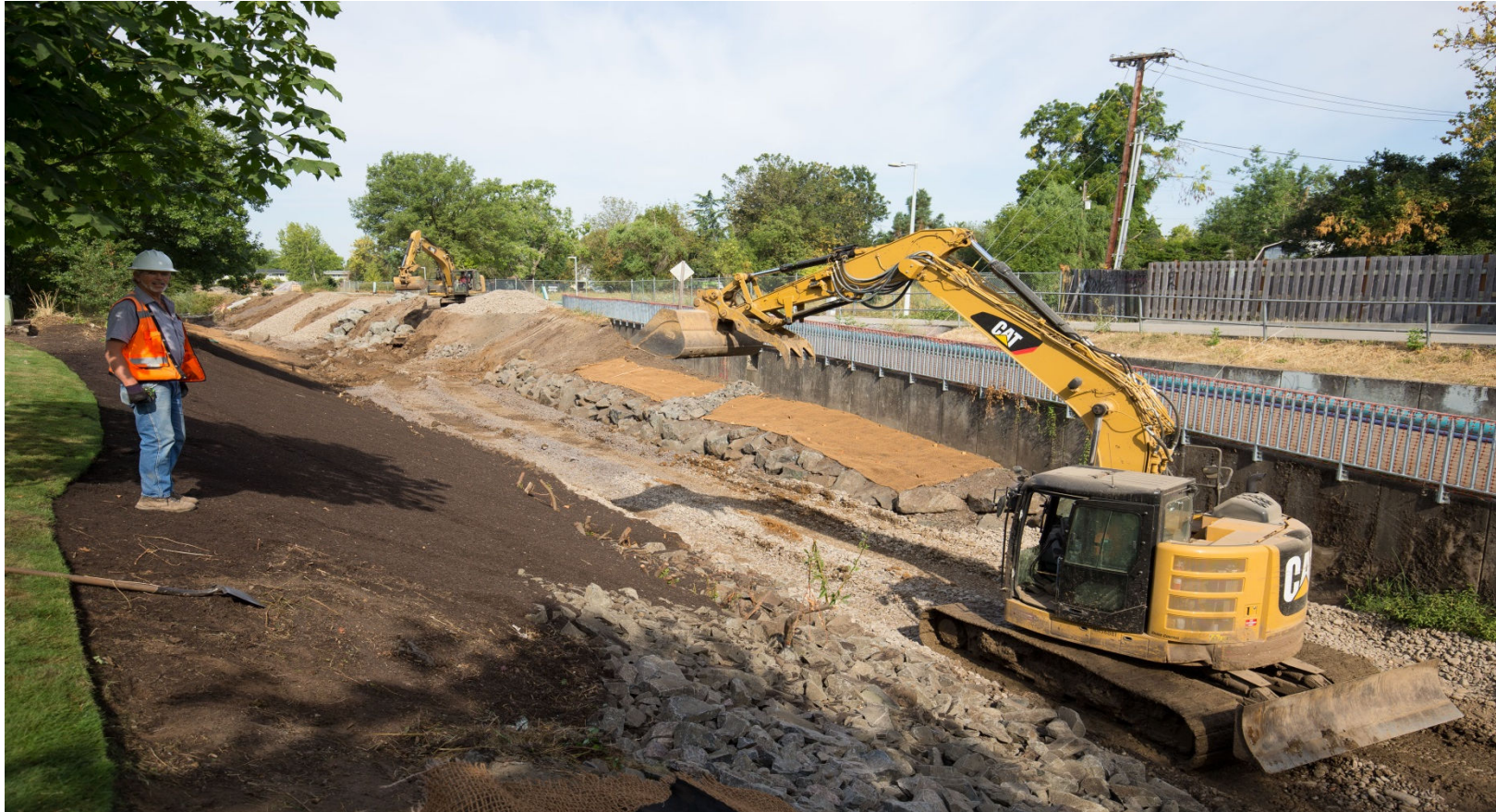
Amazon Creek Bank Capacity Improvements and Bank Stabilization
