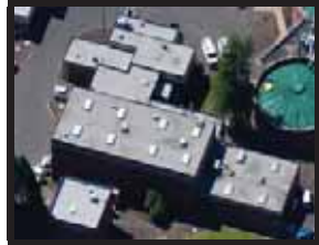
Maintenance Building Aerial
