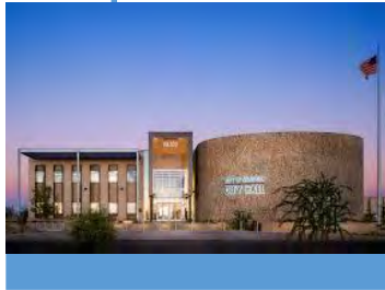
Maricopa City Hall Maricopa, AZ Completed 2013
