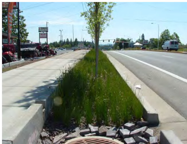
Flow-through planters serve for both landscaping and bioretention.
