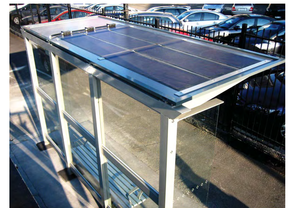
Energy Conservation -Solar Panels on Bus Stop
