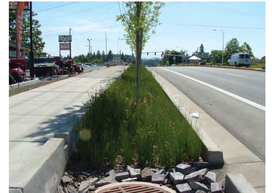
Stormwater Tretment -Flow Through Planter
