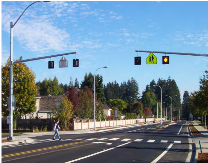
Figure 16 – Overhead Flashing Beacon
