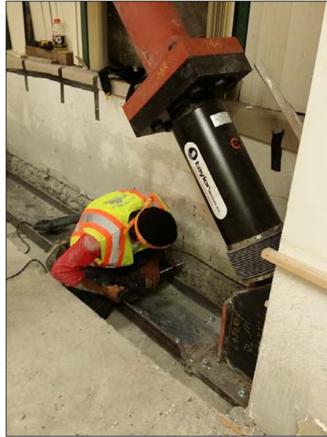
A typical damper shown above weighs about 600 lbs and is about 4' long with a 10" diameter. The damper is attached to a steel pipe with 3" thick steel plates.
