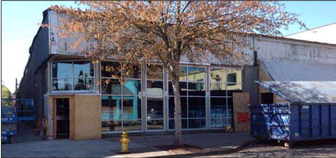
Photo: View of property from Olive Street.
