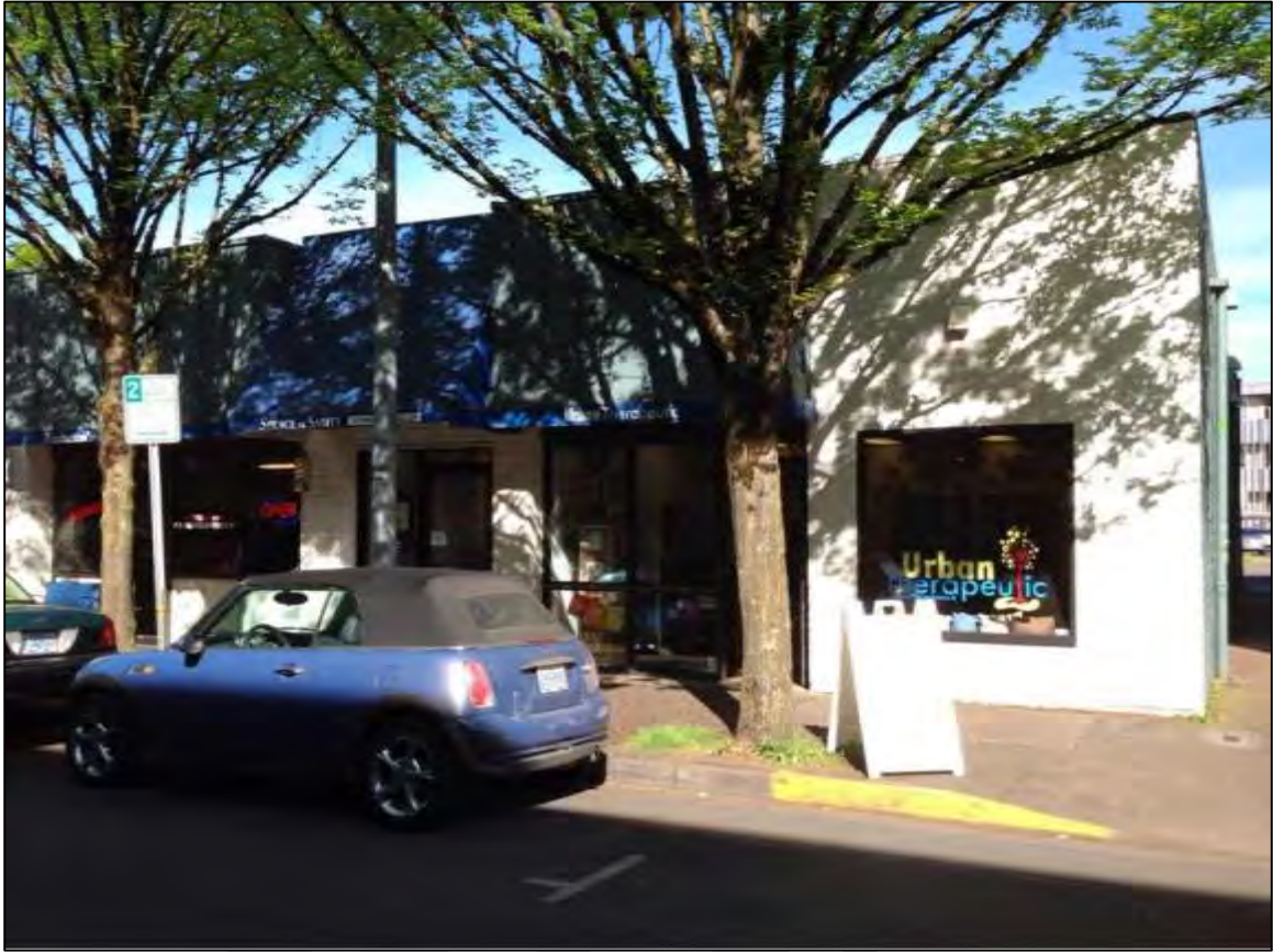
Photos: Front of building facing Willamette Street.
