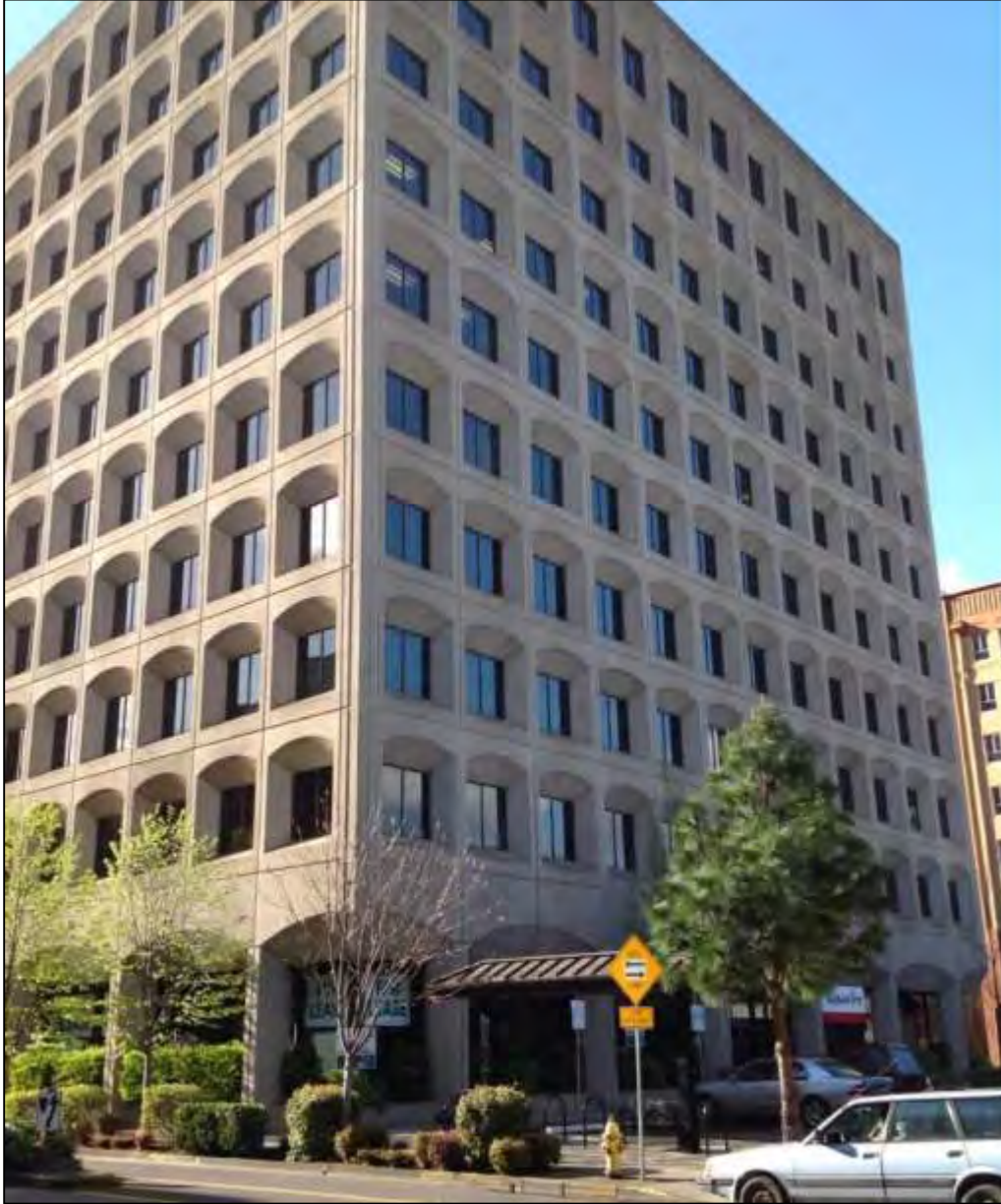
Photos: View of building on Oak Street.
