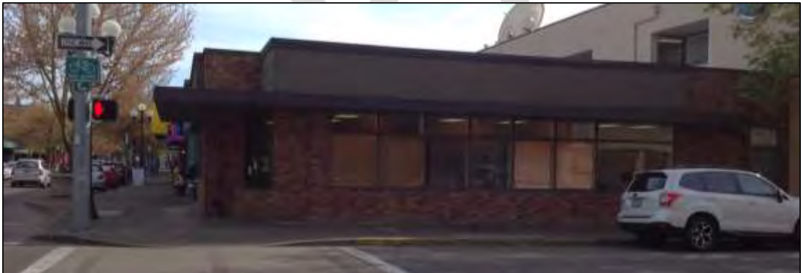
Photos: View of building on 8 th Avenue.
