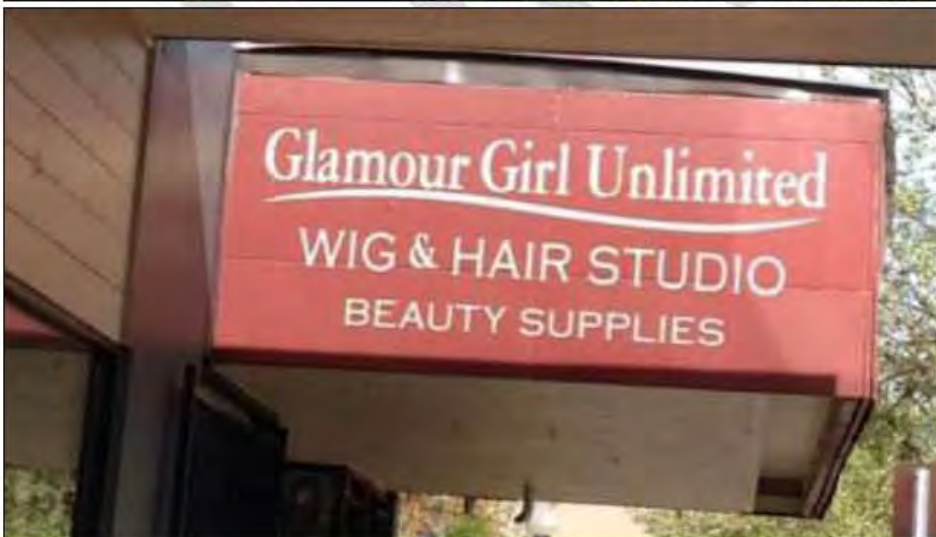
Photo: Top: view of property from Broadway; bottom: image shows damage to awning top.
