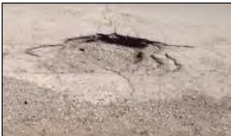
Photos: Top: front of building facing Broadway and Willamette Street; middle left: damage on building ground line; middle right: exposed pipes on building ground line; bottom: damage on parking lot.
