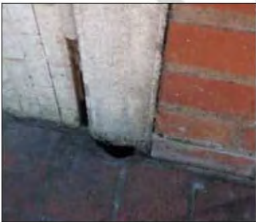
Photo: Top: View of property from Willamette Street; bottom: Damage and deterioration on front of building.
