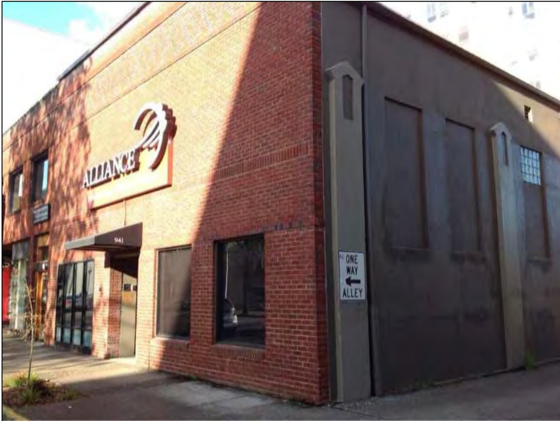
Photos: Building front facing Oak Street.
