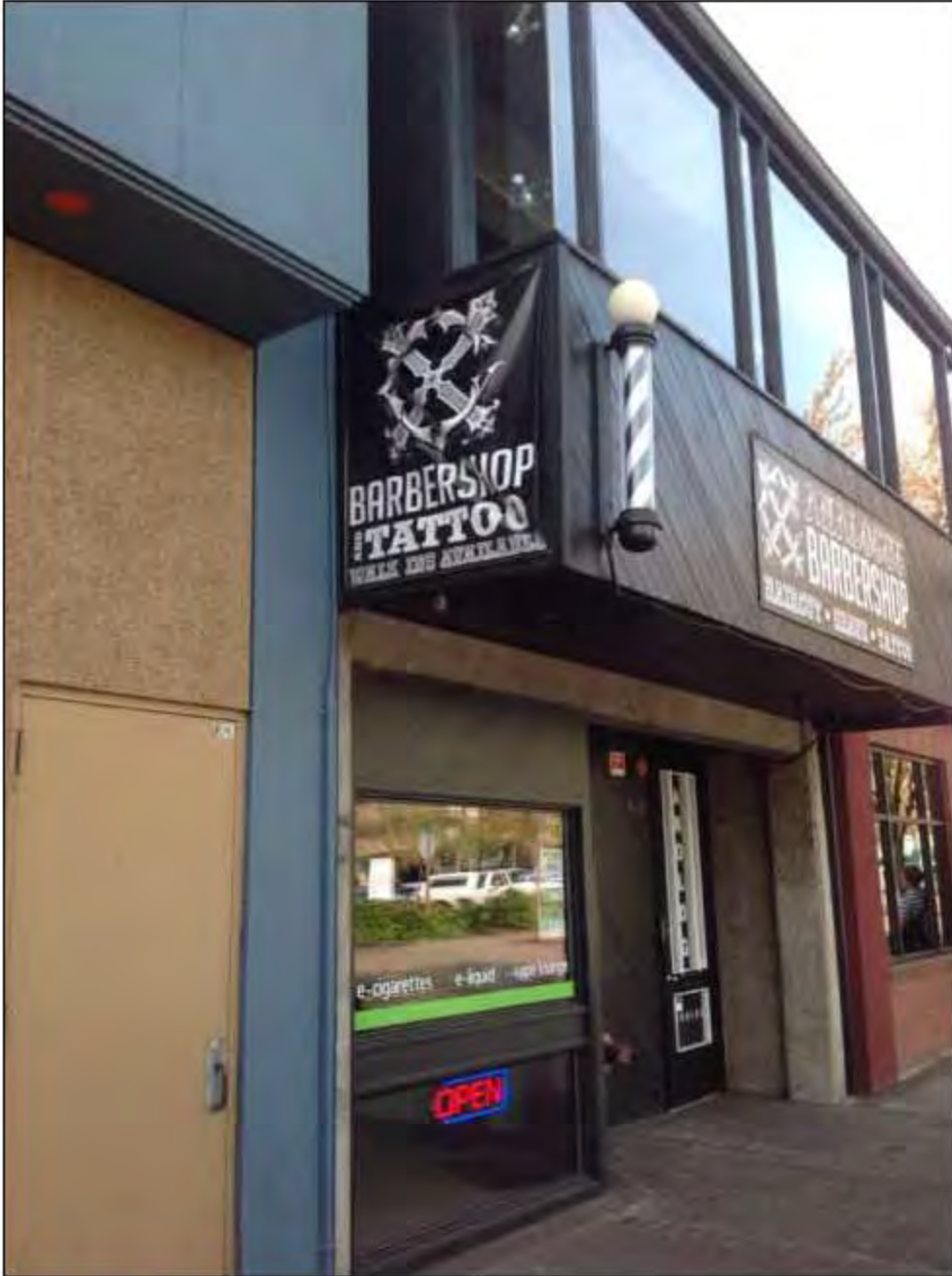
Photos: Front of building facing Olive Street.
