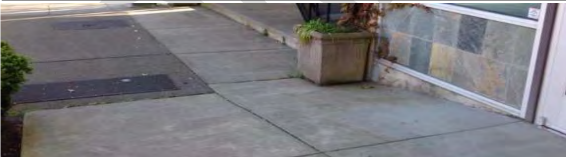
Photo: Top: view of property from Pearl Street; bottom photo shows ramp with questionable angle for accessibility.
