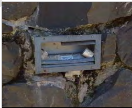
Photo: Top: view of shelter; bottom left: growth on shelter; bottom right: broken and exposed light fixture
