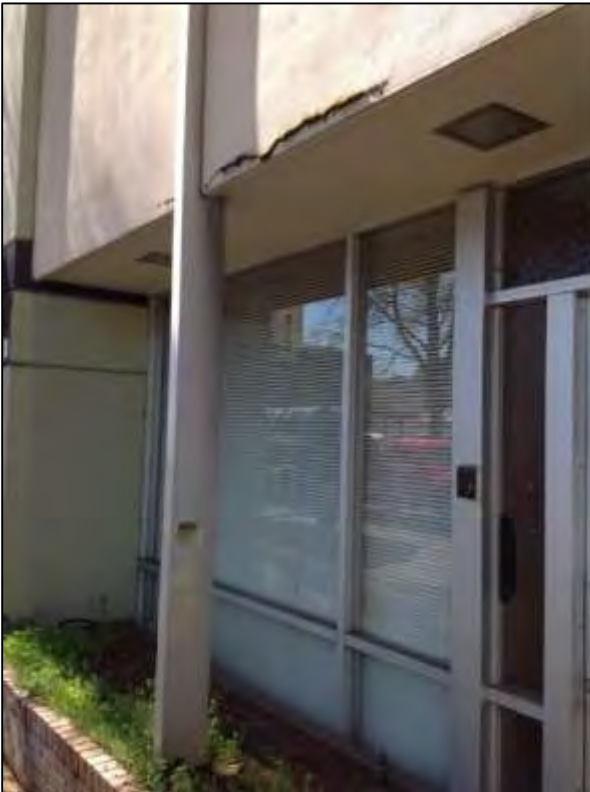
Photo: Top: damage at door base; bottom left: façade deterioration; bottom right: broken bricks, overgrown vegetation.
