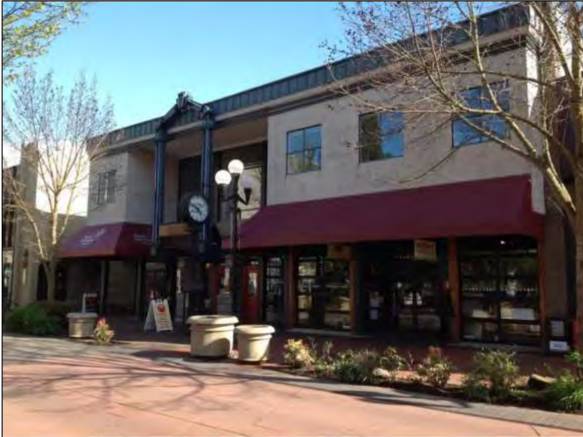
Photos: Building front facing East Broadway.
