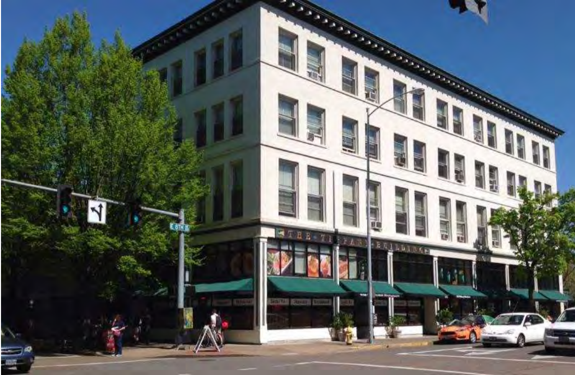
Photo: View of property from Willamette Street and East 8 th Avenue.
