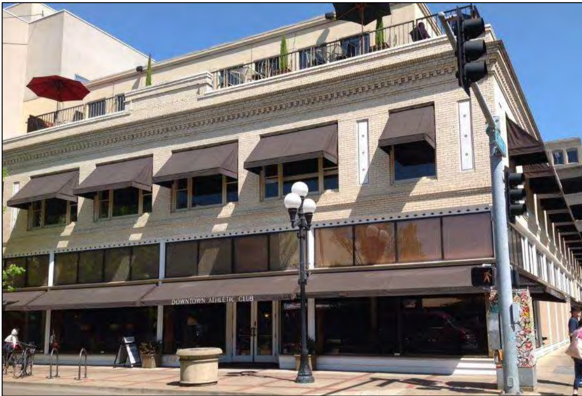
Photos: View of property from East 10 th Avenue and Willamette Street.
