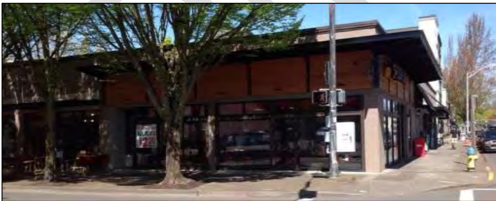
Photos: Top: view of property along East Broadway; bottom: view of building from East Broadway and Pearl Street.
