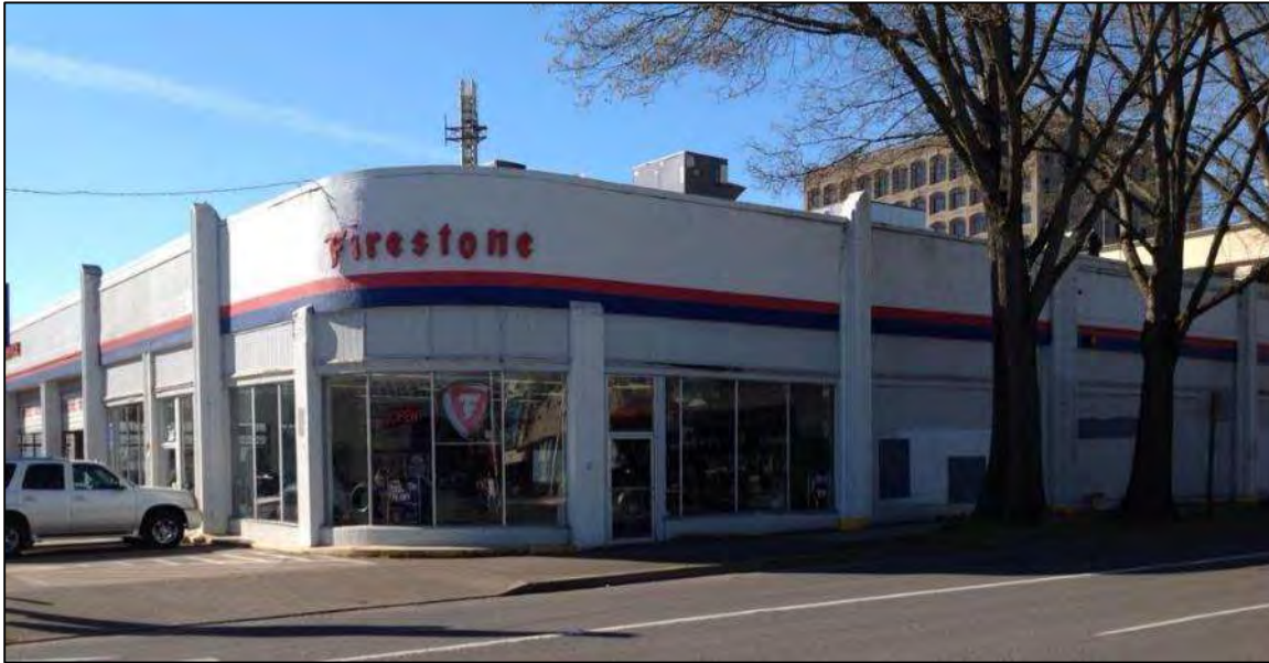
Photo: View of property from East 11 th Avenue and Pearl Street.
