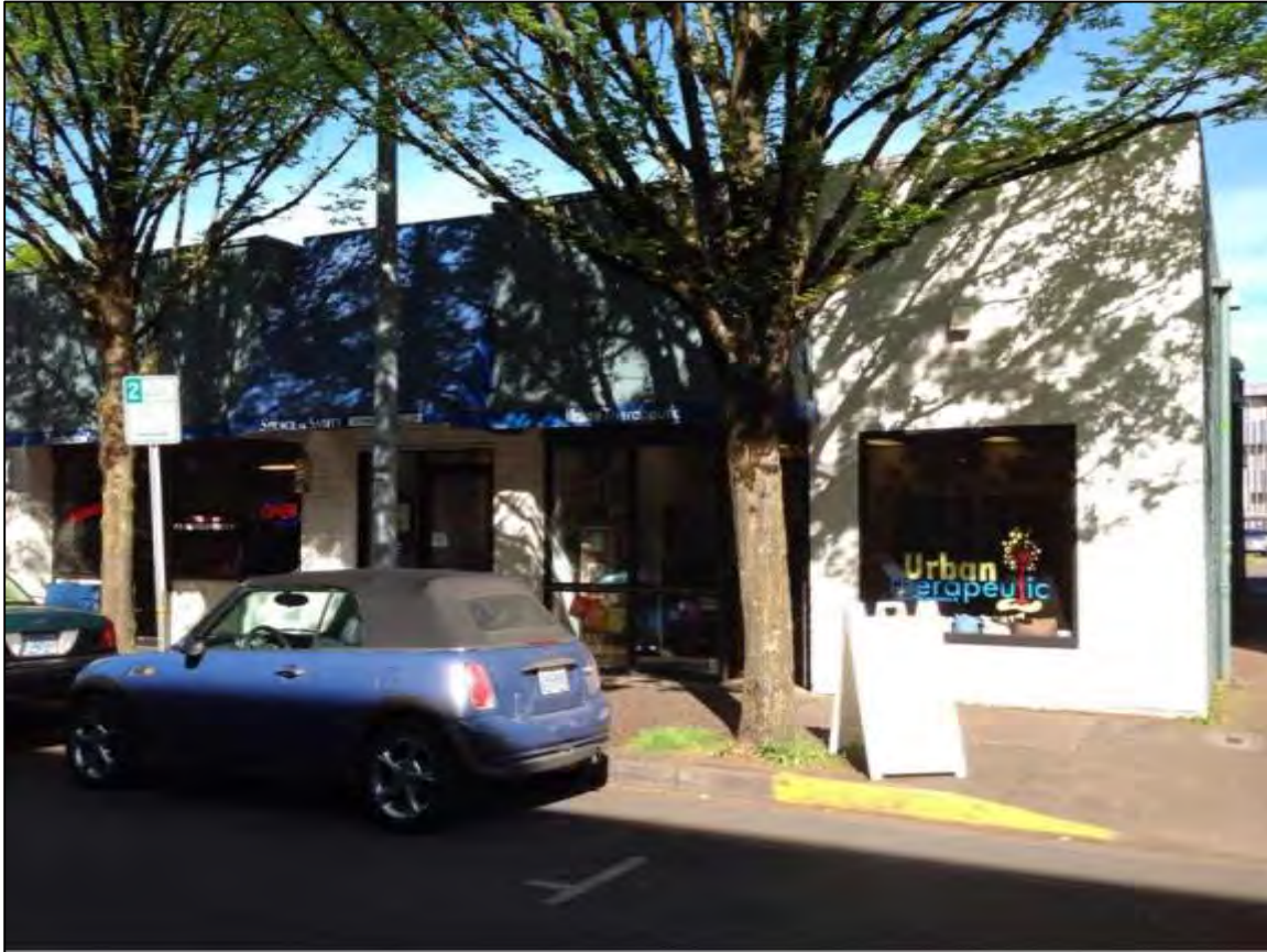
Photos: Front of building facing Willamette Street.
