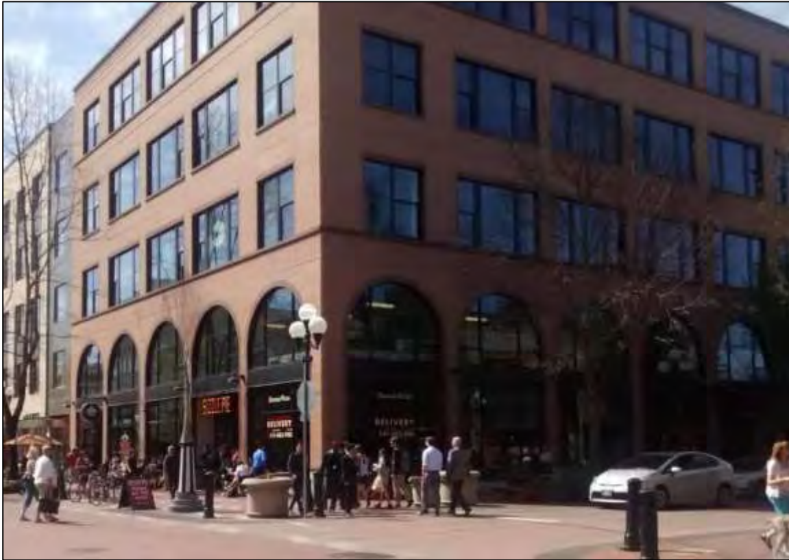
Photos: View of building on Broadway and Willamette Street.
