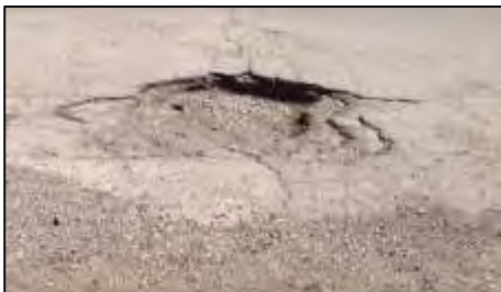
Photos: Top: front of building facing Broadway and Willamette Street; middle left: damage on building ground line; middle right: exposed pipes on building ground line; bottom: damage on parking lot.
